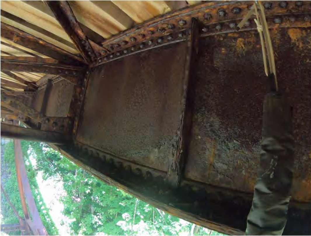
59. Very Severe Corrosion and Forty Percent Section Loss of Vertical Web Stiffener
