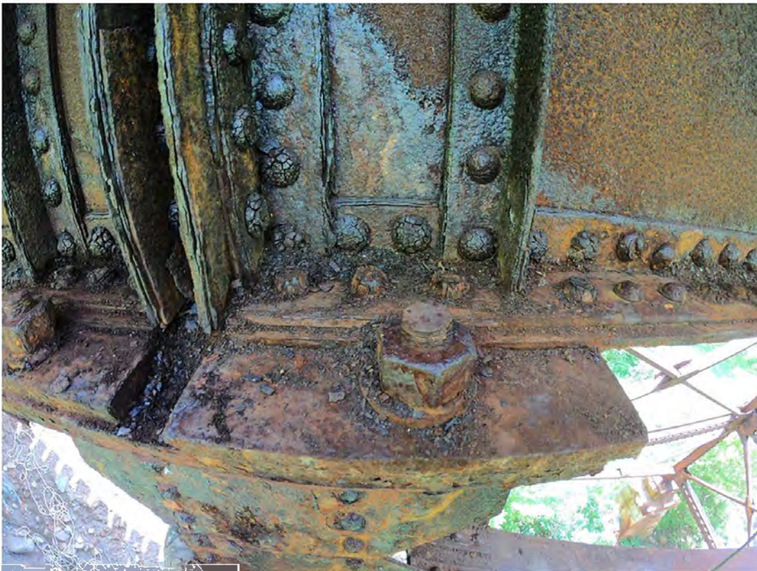
16. Medium Corrosion of Bearing Plate
