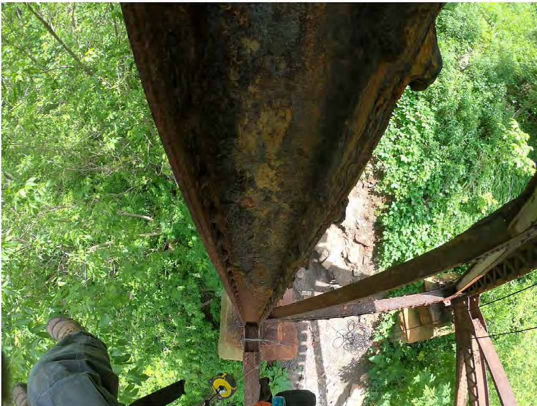
20. Medium Corrosion and Delamination on Column
