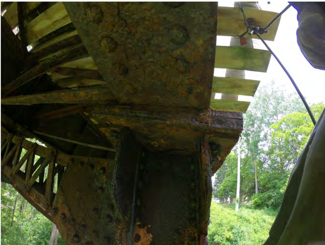
40. Medium Corrosion and Delamination of Bearing Plate at Girder; Medium Corrosion and Delamination on Bottom Flange of Girder
