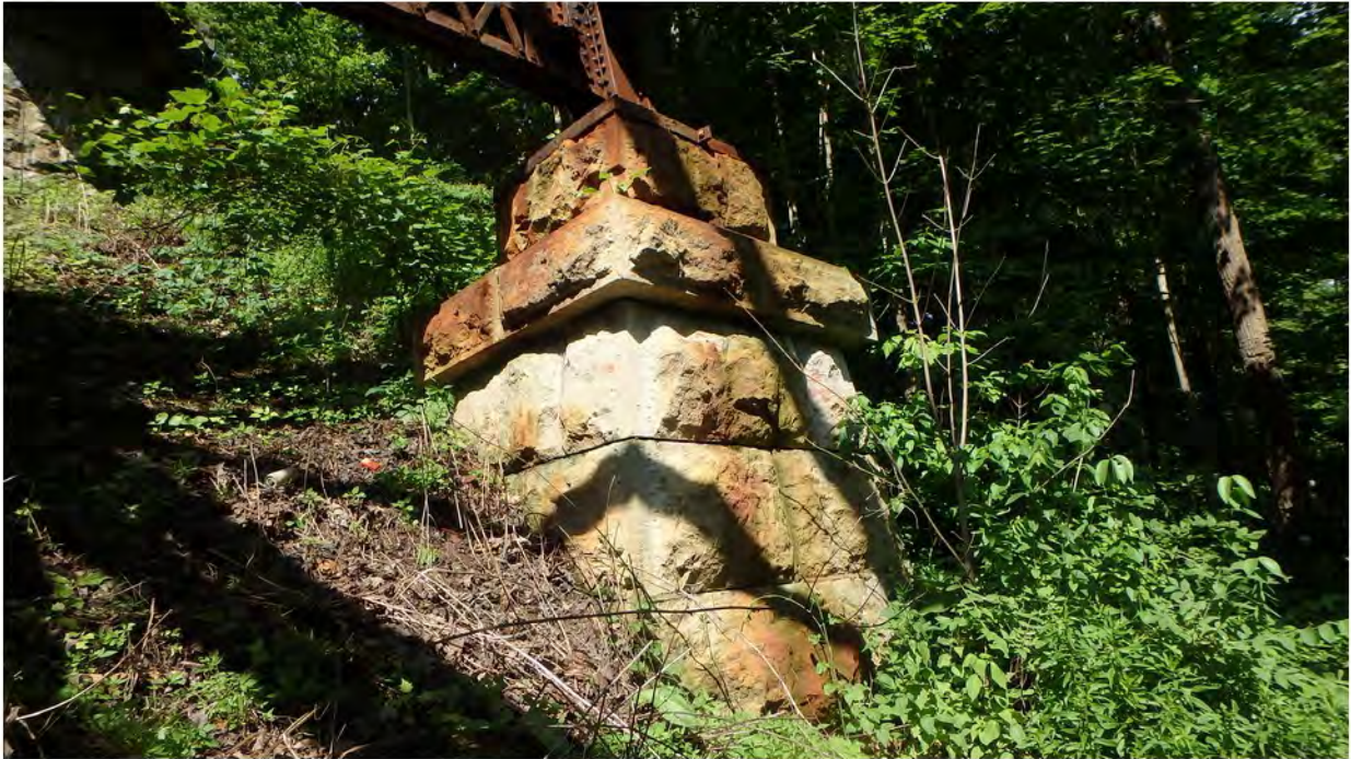
77. Staining and Vertical Cracking in Bearing Block; Staining in North B Pier
