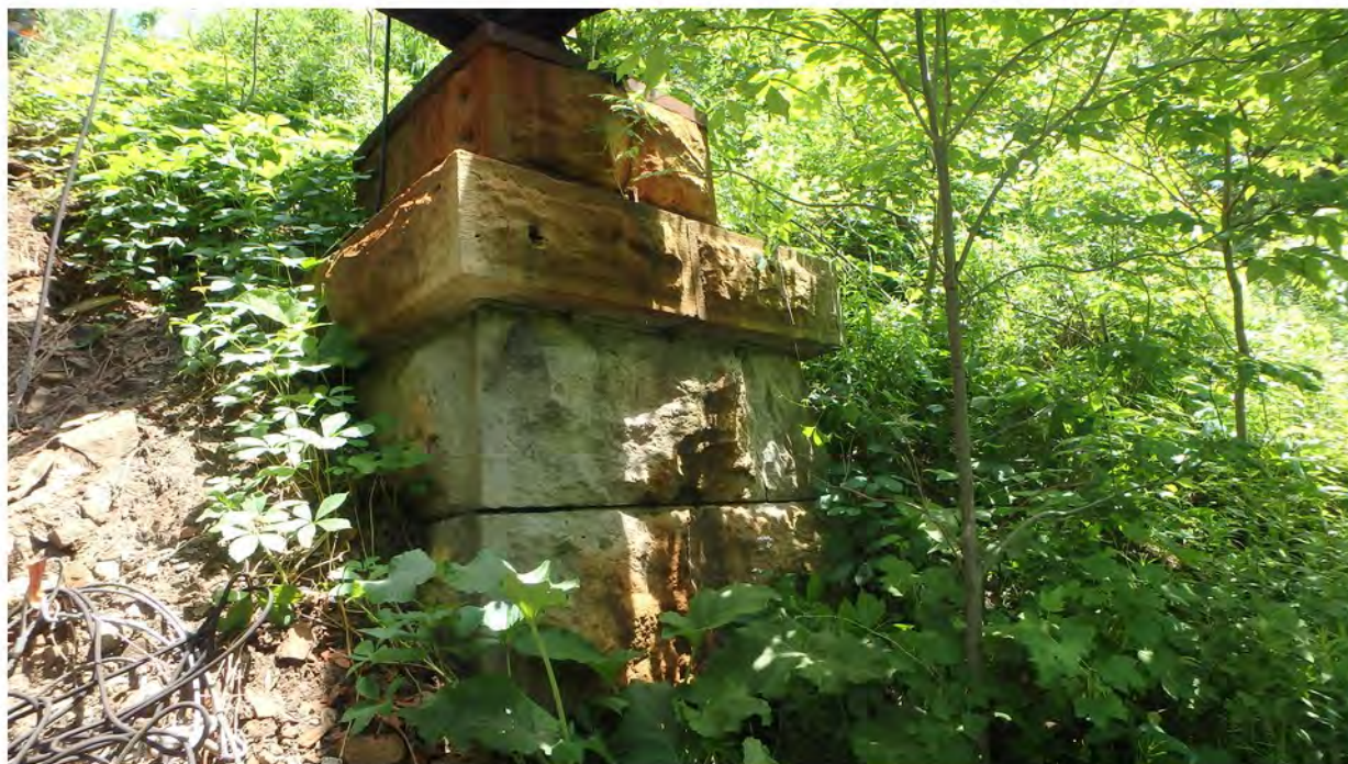
93. South I Pier; Staining Typical
