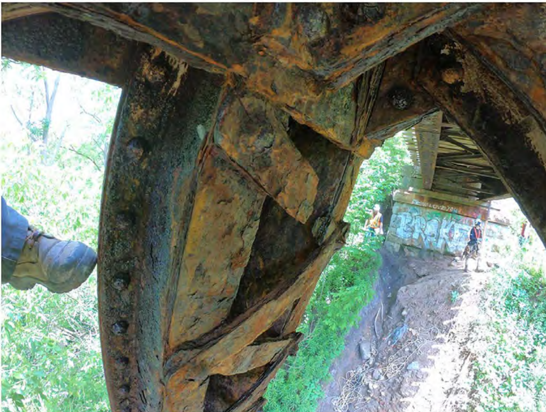
18. Very Severe Corrosion and Delamination with Complete Section Loss on Column Brace
