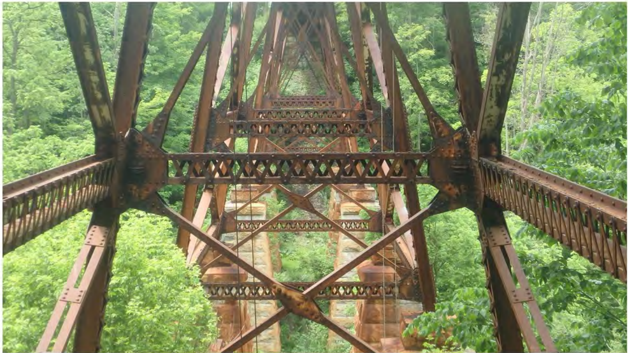
71. Medium to Severe Corrosion on Lateral Supports
