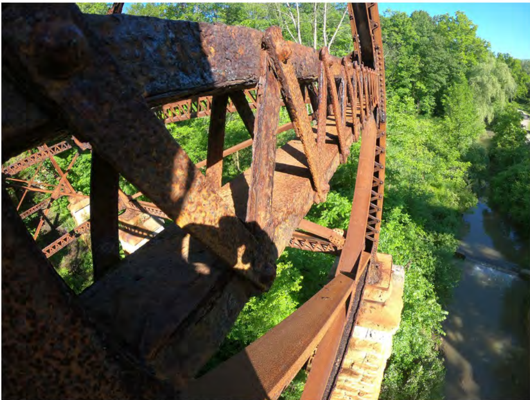
54. Severe Corrosion of Lateral Support and Lace Bracing at Centre of Columns, Typical
