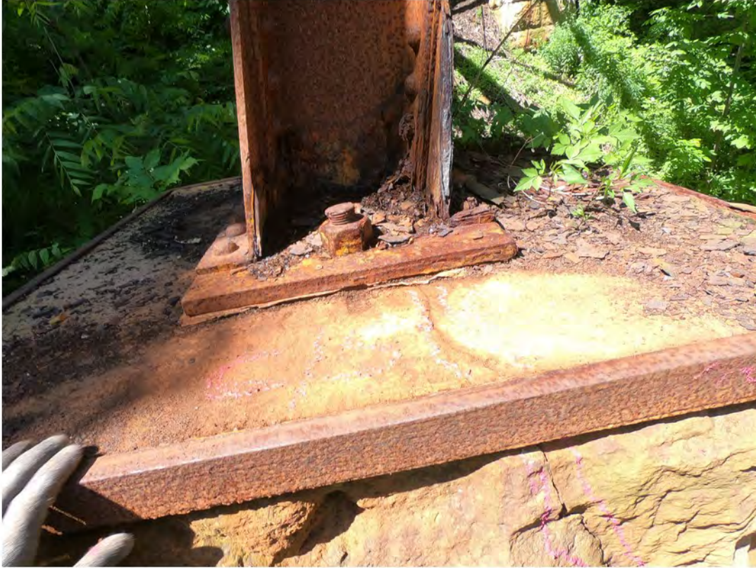
61. Vertical Crack in Bearing Block; Severe Corrosion of Column at Connection
