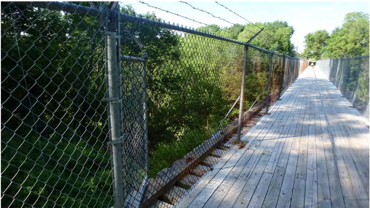
102. Light Corrosion on Fence at Both Sides of Deck, Typical
