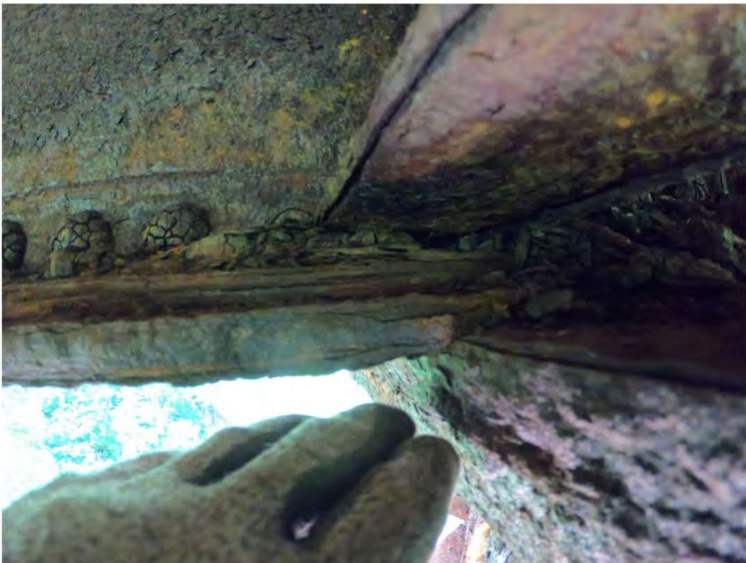
36. Deterioration of the Girder Flange at the South H Column
