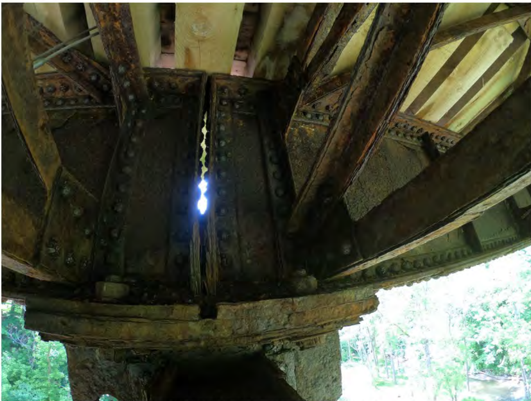
38. Severe Corrosion and Delamination of Diaphragm; Medium Corrosion and Delamination of Girder and Bearing Plate
