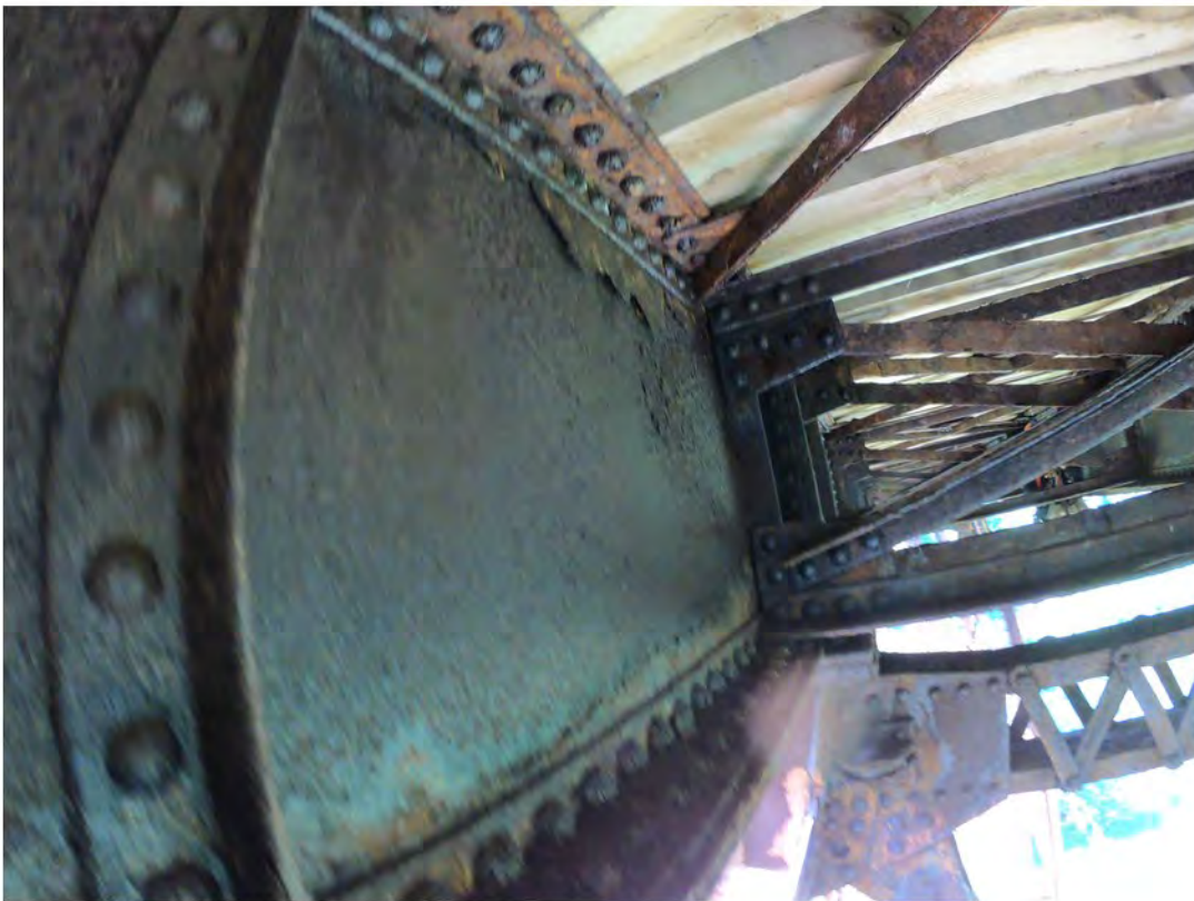
34. Medium Corrosion and Delamination of Girder
