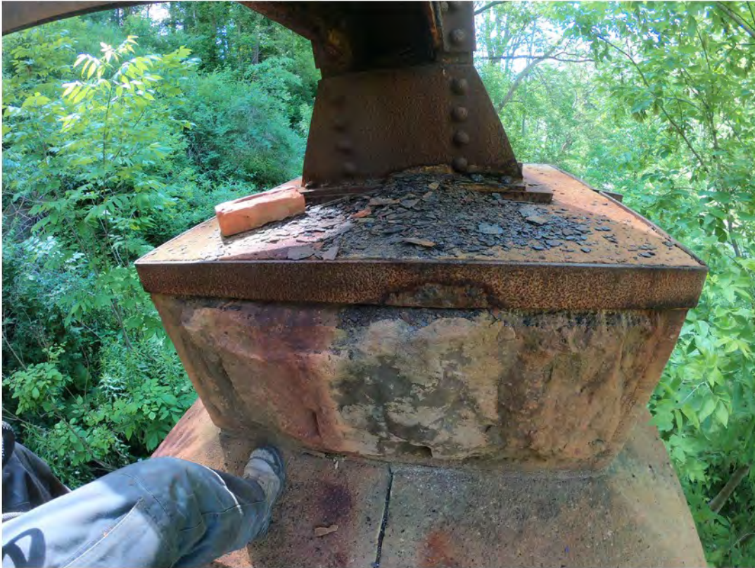
31. Medium Corrosion of Bearing Plate; Staining of Pier Cap
