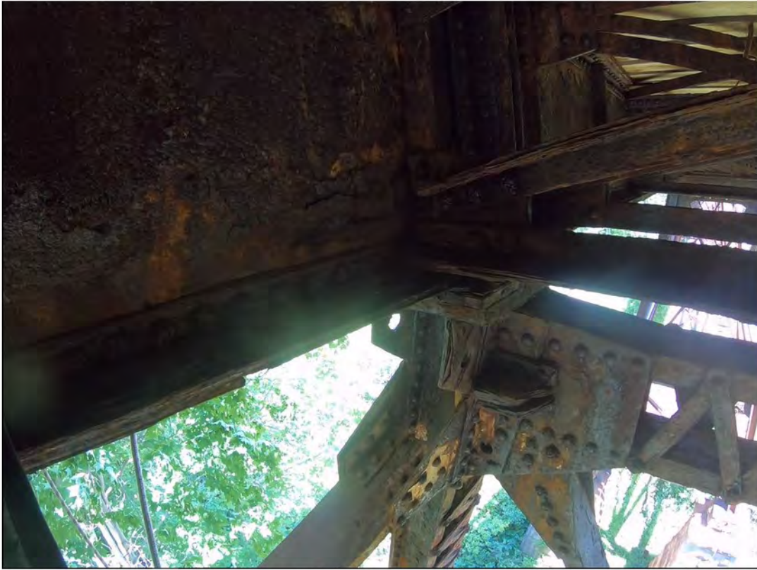
67. Very Severe Corrosion and Fifty Percent Section Loss of Bracket Under Bearing Seat
