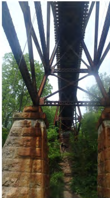
71. Medium to Severe Corrosion on Lateral Supports
