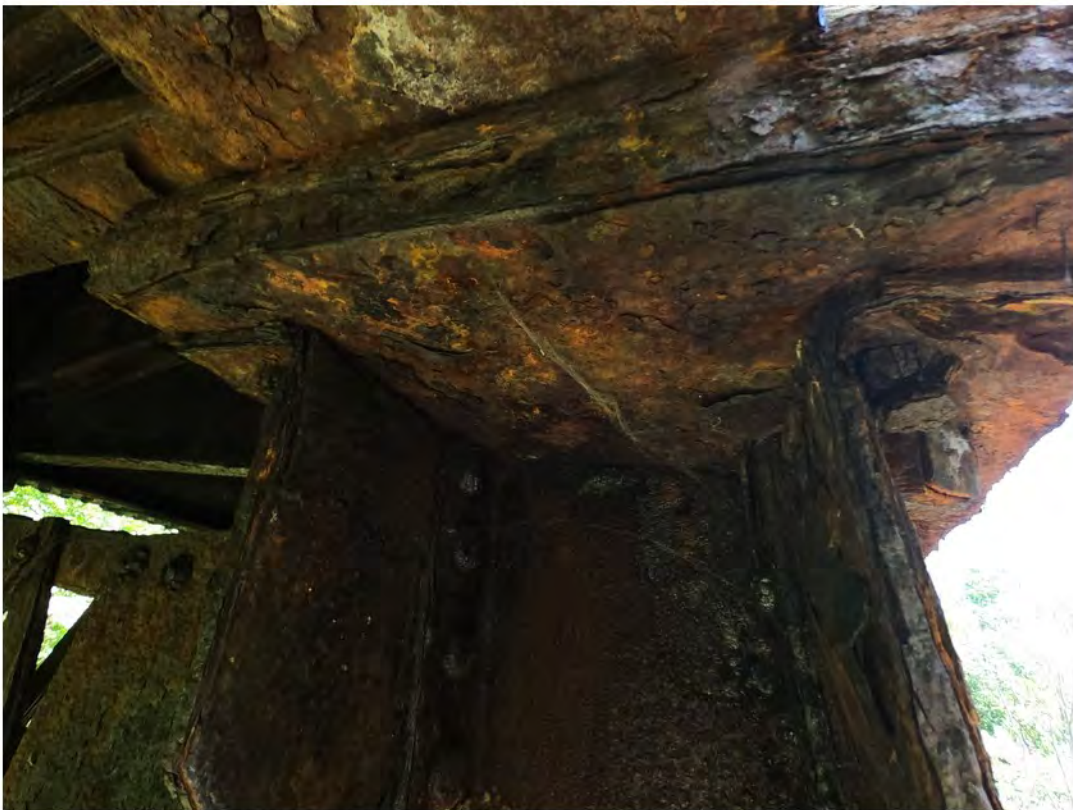
68. Severe Corrosion and Delamination at Connection Between Column and Girder
