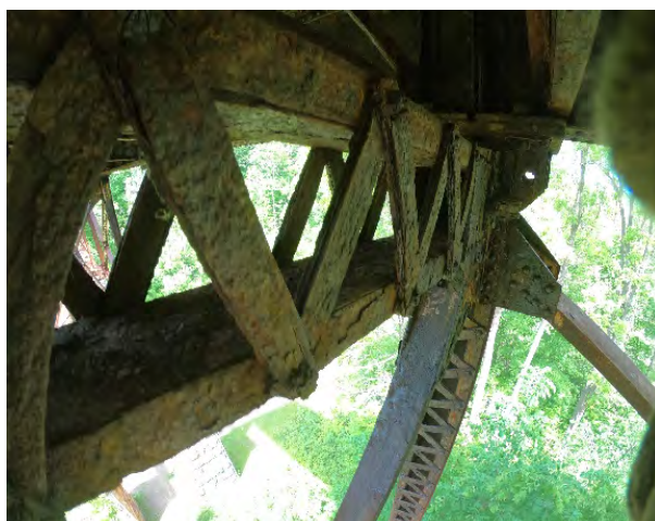
Figure 3 & 4: Severely Deteriorated Laces Bracing throughout, Note Broken Brace in Figure 3
