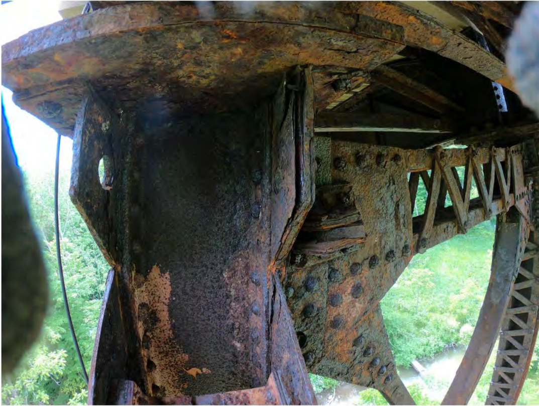
45. Very Severe Deterioration and Delamination of Bearing Seat at Top of Column
