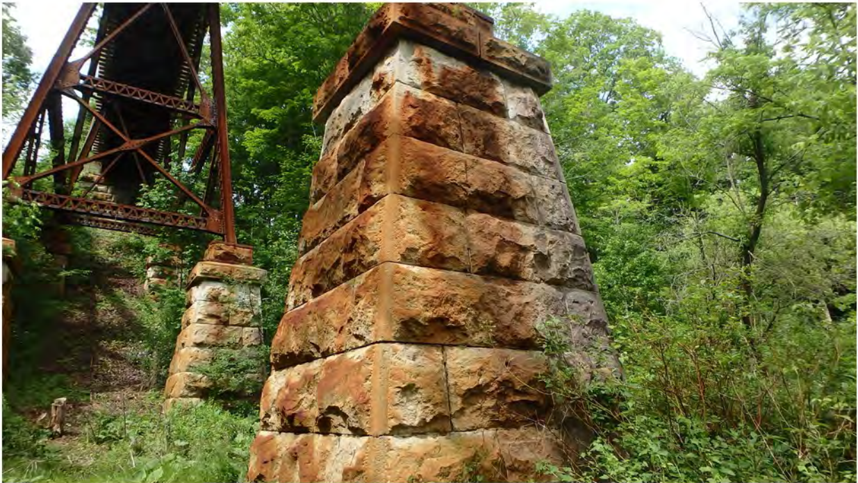
81. North D Pier; Staining Throughout
