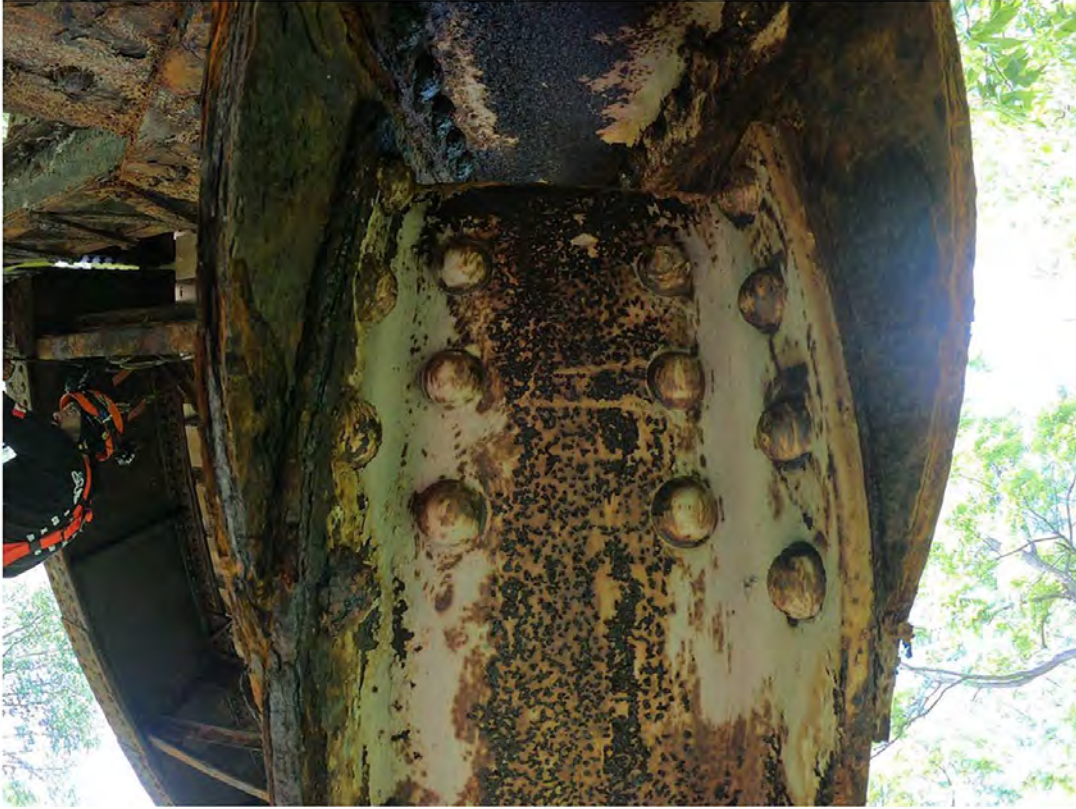
21. Medium Corrosion of Column at Girder
