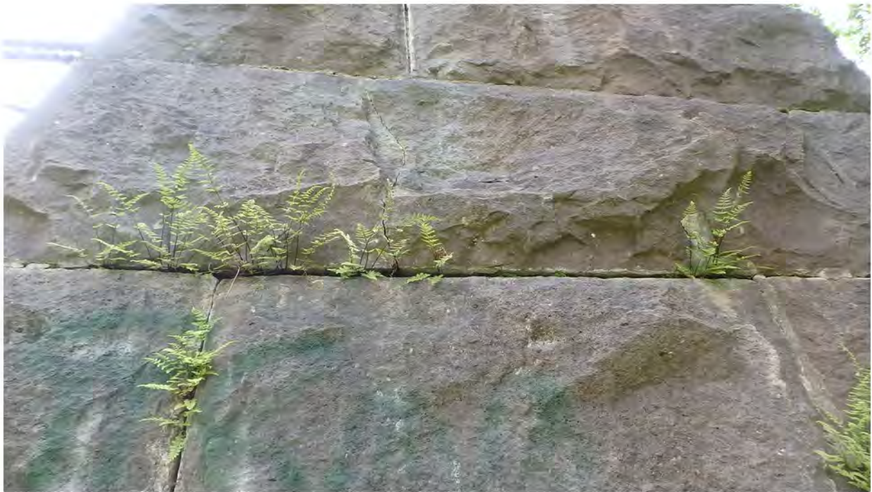
95. Cracking and Mortar Loss on Piers, Typical
