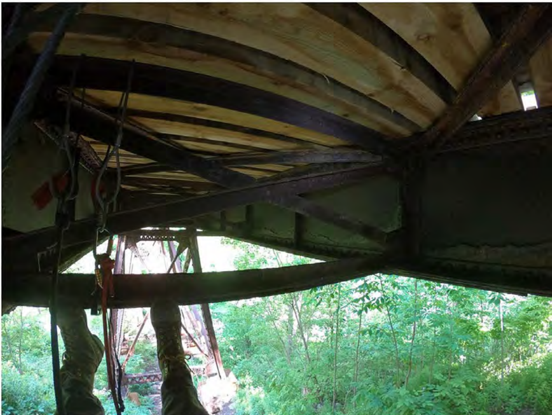
8. Severe Corrosion and Delamination on Girder and Diaphragm
