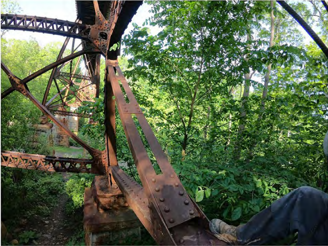
7. Surface Corrosion on Diagonal Bracing, Typical
