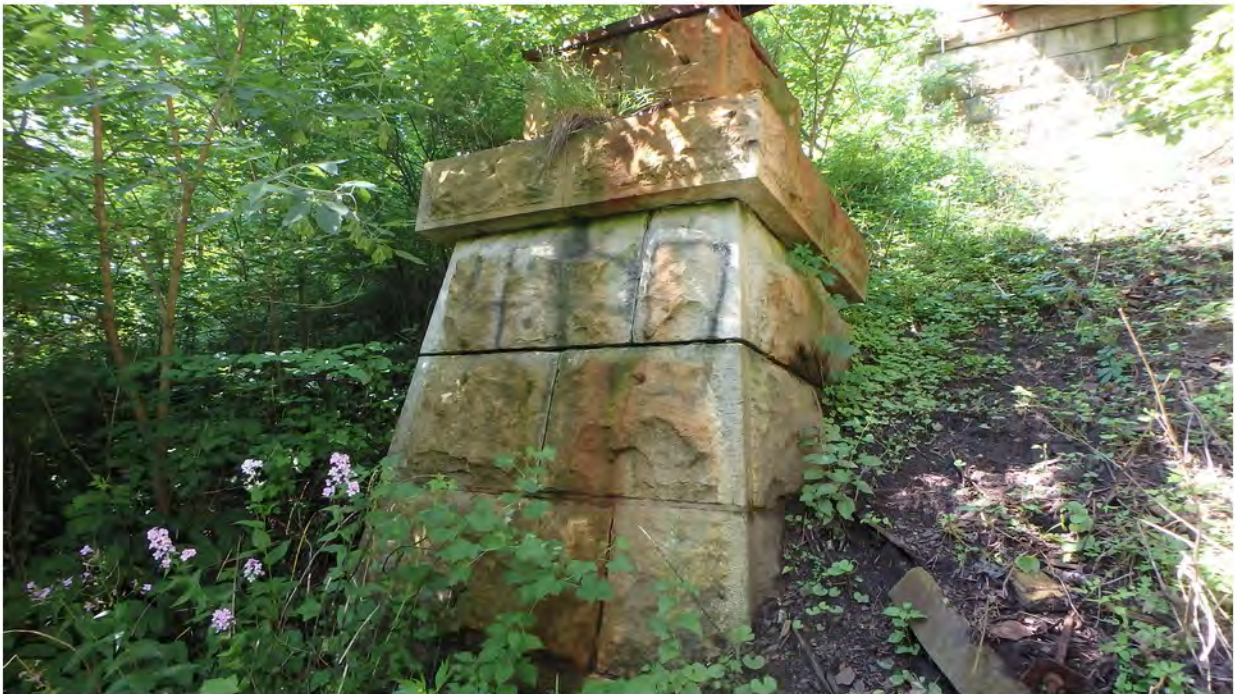
76. Vertical Cracking in Bearing Block; Separation of Concrete Blocks in South B Pier
