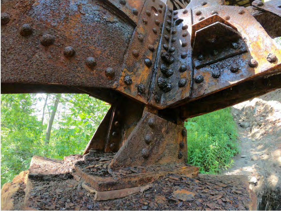
25. Medium Corrosion on Bearing Plate, and Surrounding Members; Cracking of Rivets
