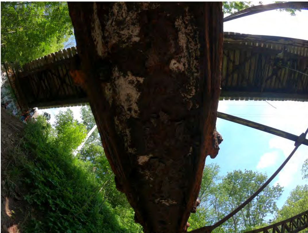
24. Severe Corrosion and Delamination of Bottom Horizontal Chord
