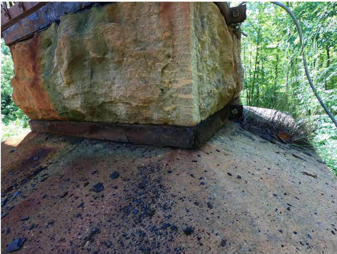
58. Medium Corrosion and Delamination of Steel Between Pier and Pier Cap
