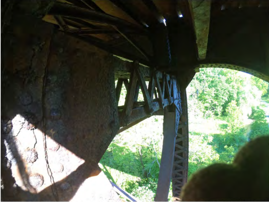
51. Severe Corrosion and Delamination of Connections and Cracking of Rivets at Lateral Support
