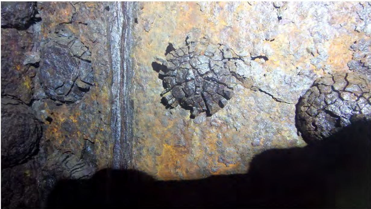
66. Rivet Cracking; Typical Throughout Structure
