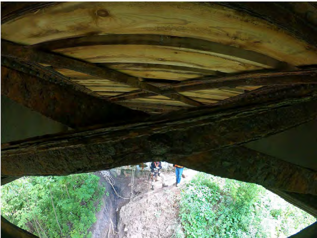
12. Severe Corrosion and Delamination of Diagonal Components of Diaphragm
