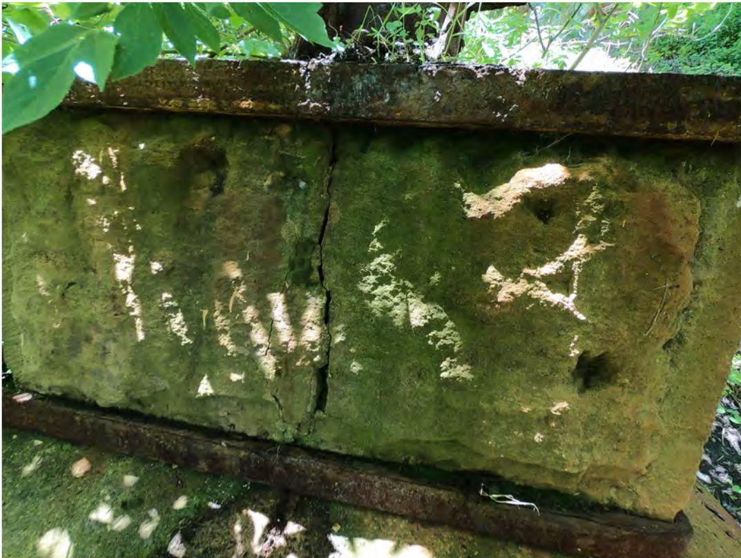
64. Vertical Cracking Through Pier Cap
