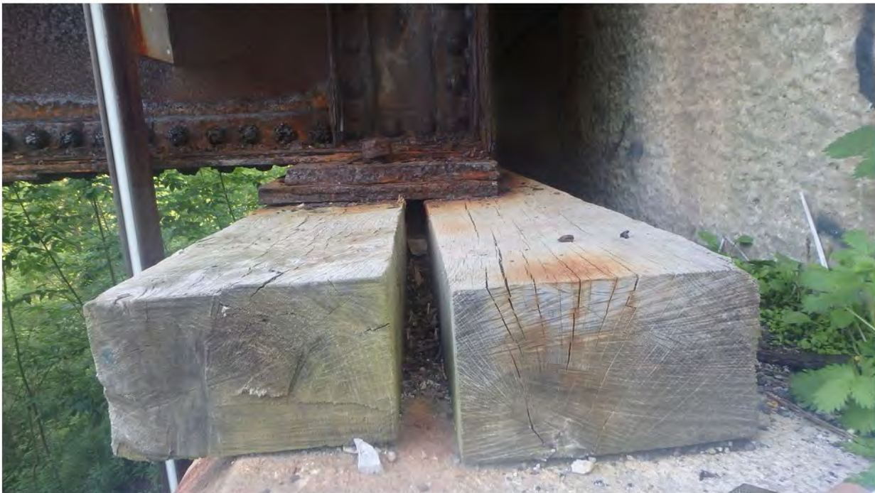
70. Minor Checks and Shakes in Wood at East Abutment
