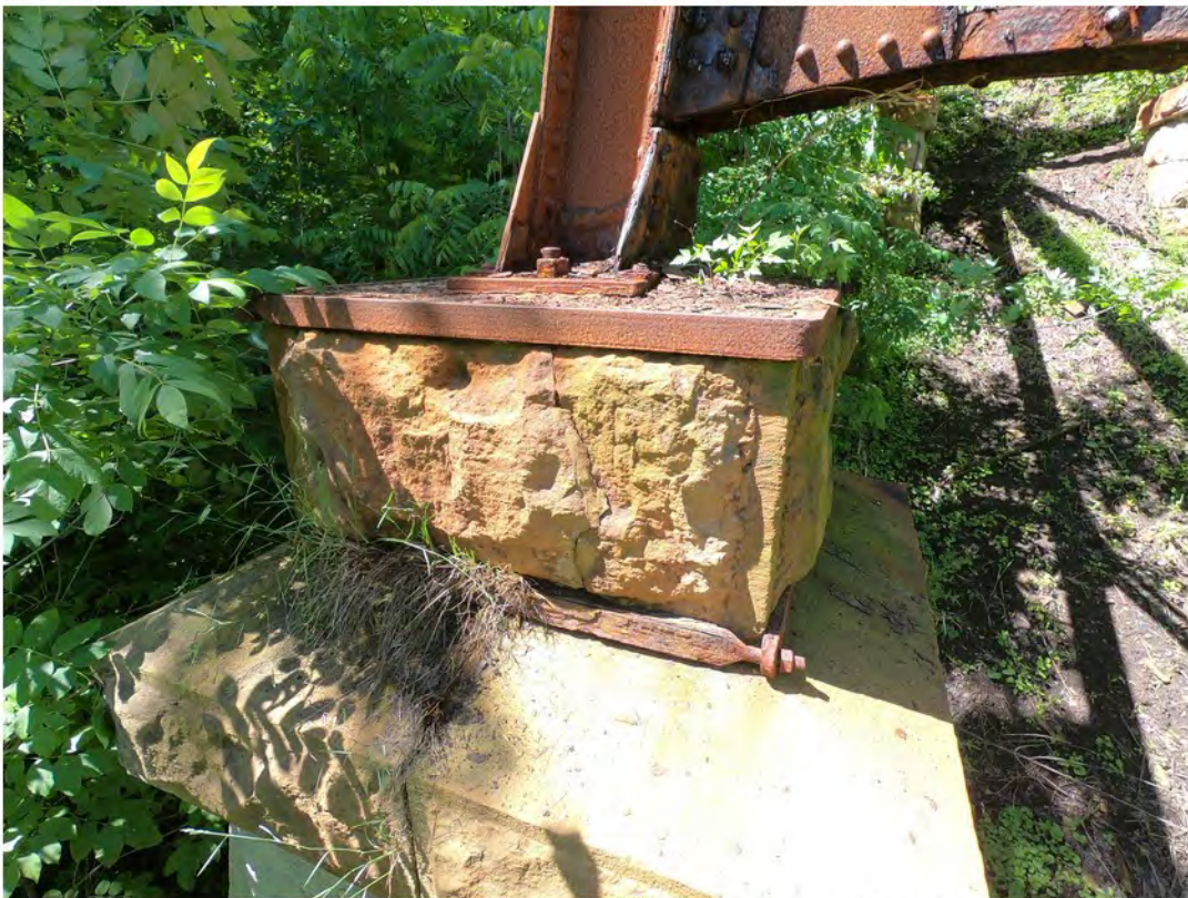
60. Severe Corrosion and Delamination of Steel at Bottom of Pier Cap; Vertical Crack in Pier Cap
