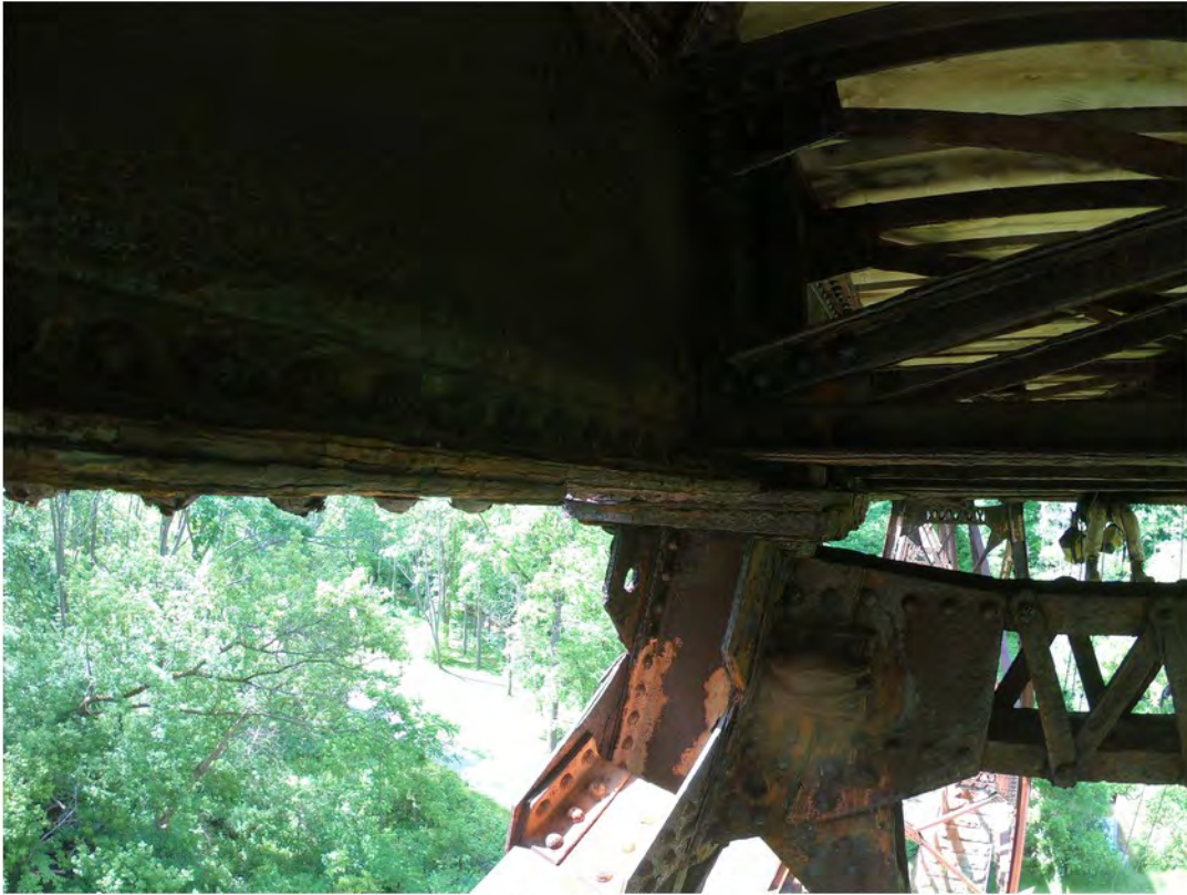
33. Medium Corrosion of Girder; Cracking of Rivets and Delamination of Bottom Flange
