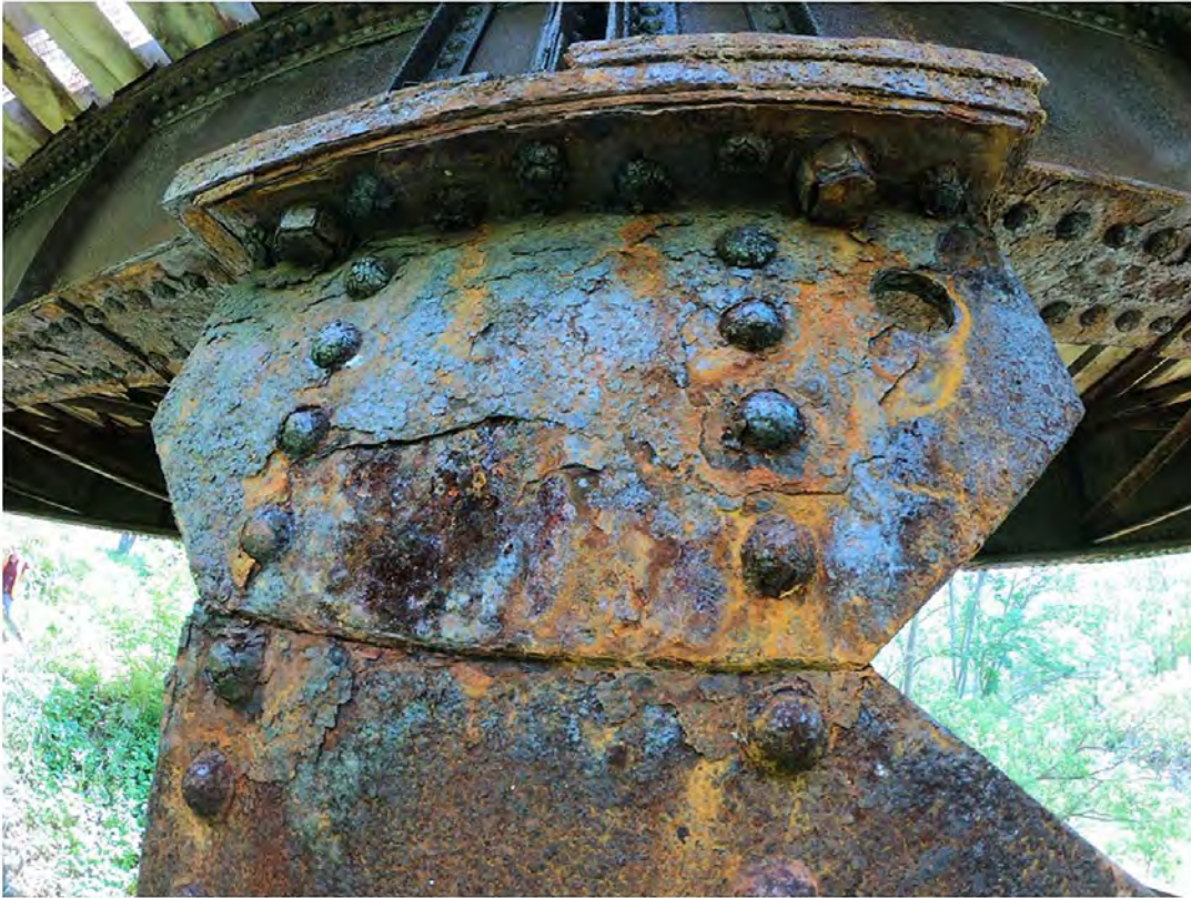
17. Medium Corrosion and Delamination of Connection Plate at Column End
