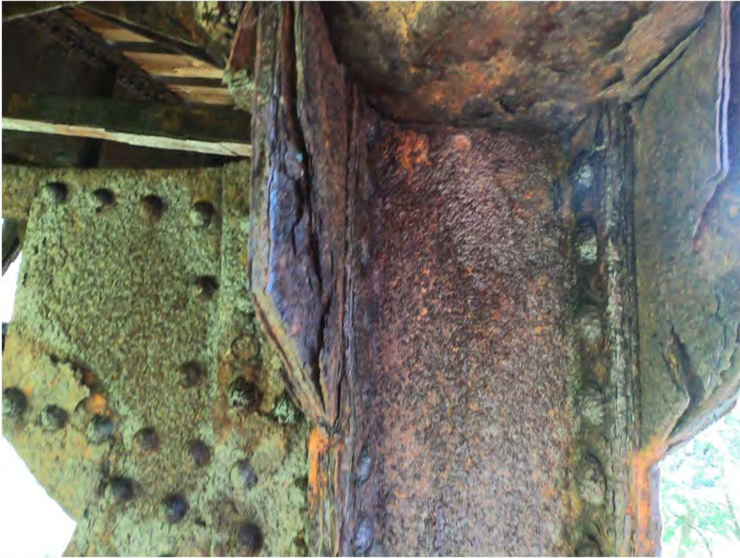
57. Severe Corrosion and Delamination at Connection of Column to Girder
