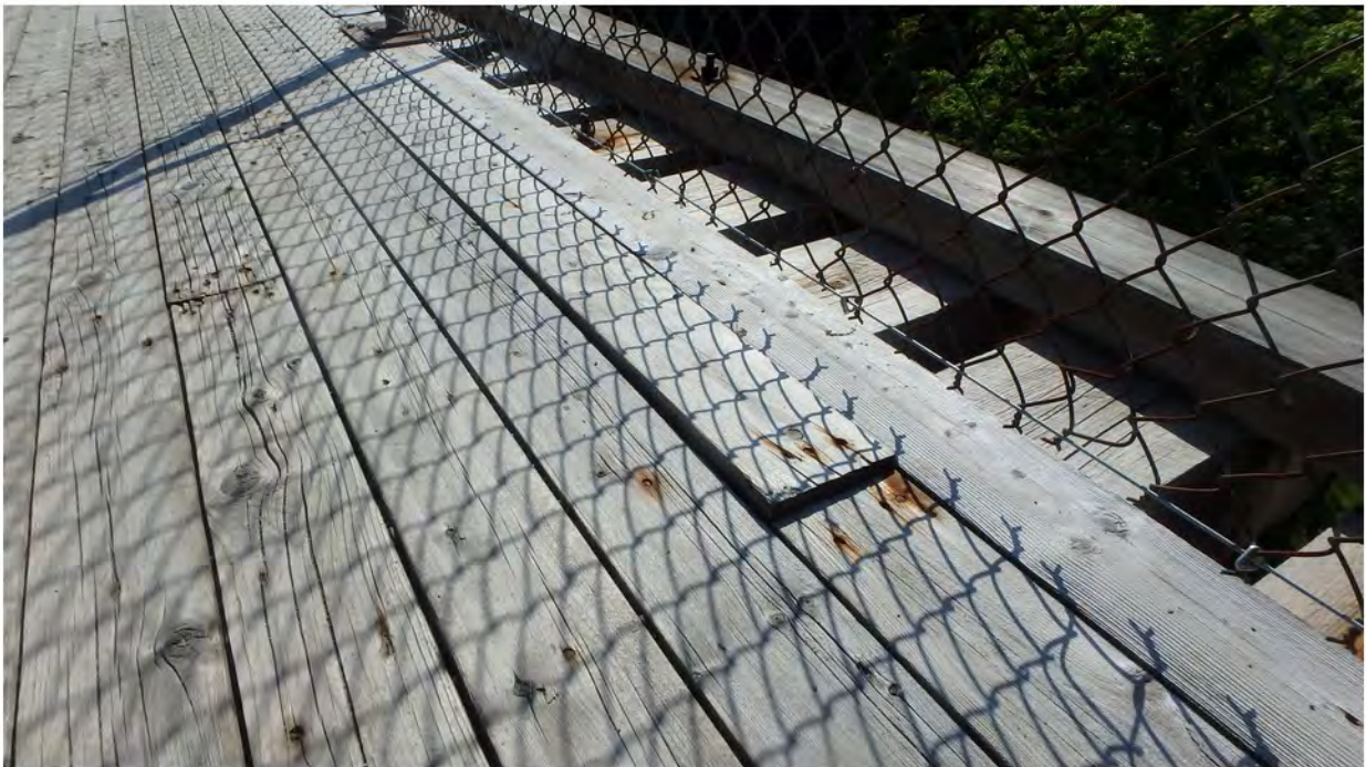
104. Lifting of Deck Boards Along Deck Wearing Surface
