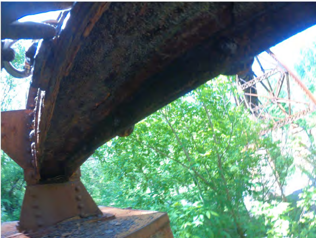
32. Severe Corrosion and Delamination of Bottom Horizontal Chord of Lateral Support
