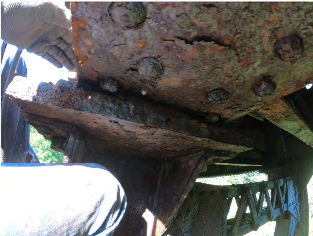
52. Severe Corrosion and Delamination on Bottom Flange of Girder at Column Connection
