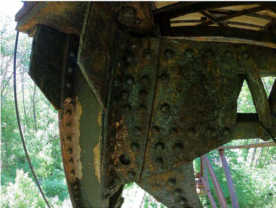
14. Severe Corrosion and Delamination on Columns
