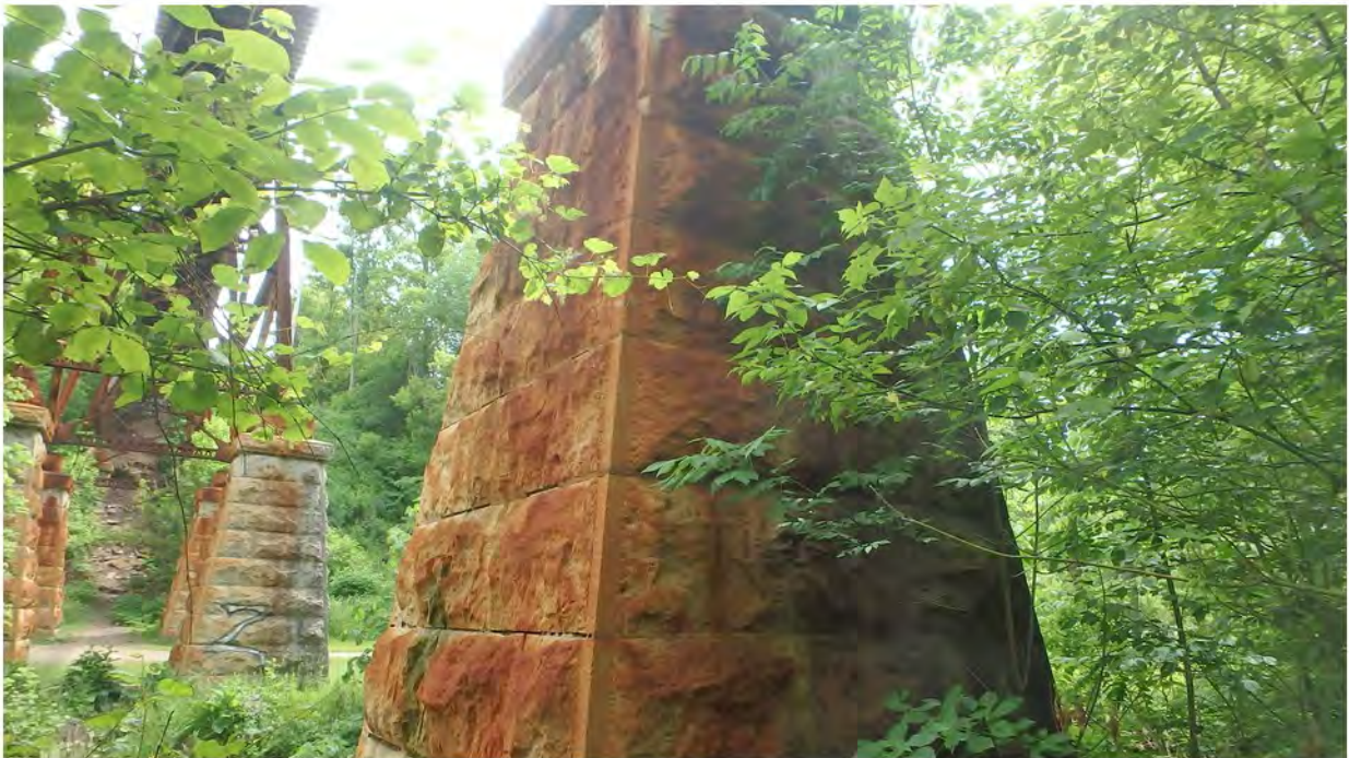
80. South D Pier; Staining Throughout
