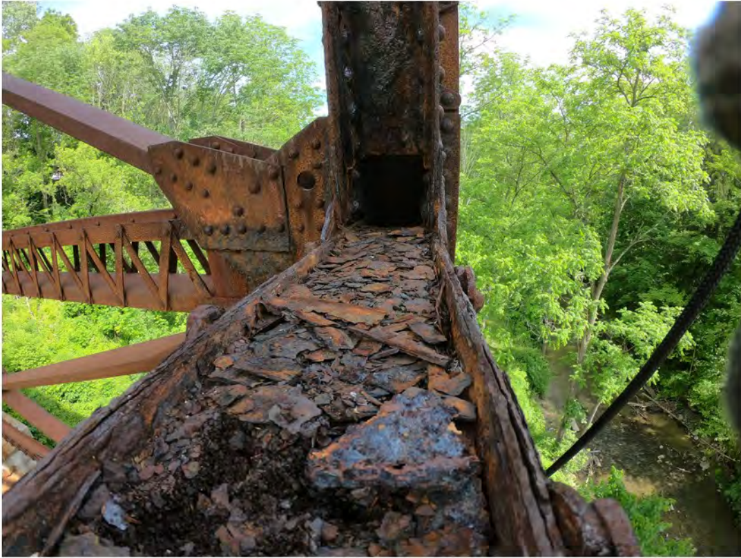
47. Very Severe Corrosion and Delamination of Horizontal Chord
