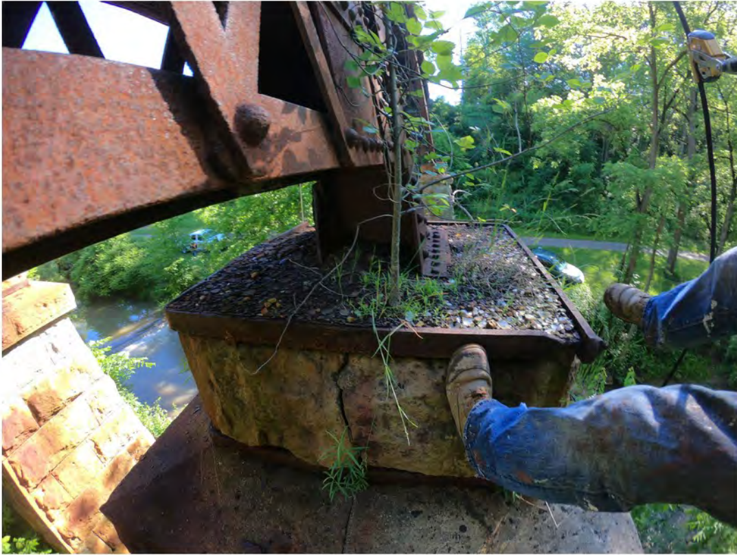
55. Medium Corrosion of Connection Between Column and Bearing Seat; Vertical Crack in Pier Cap
