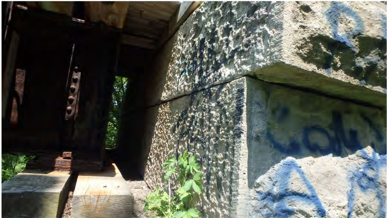
99. South East Bearing; Medium Corrosion and Delamination
