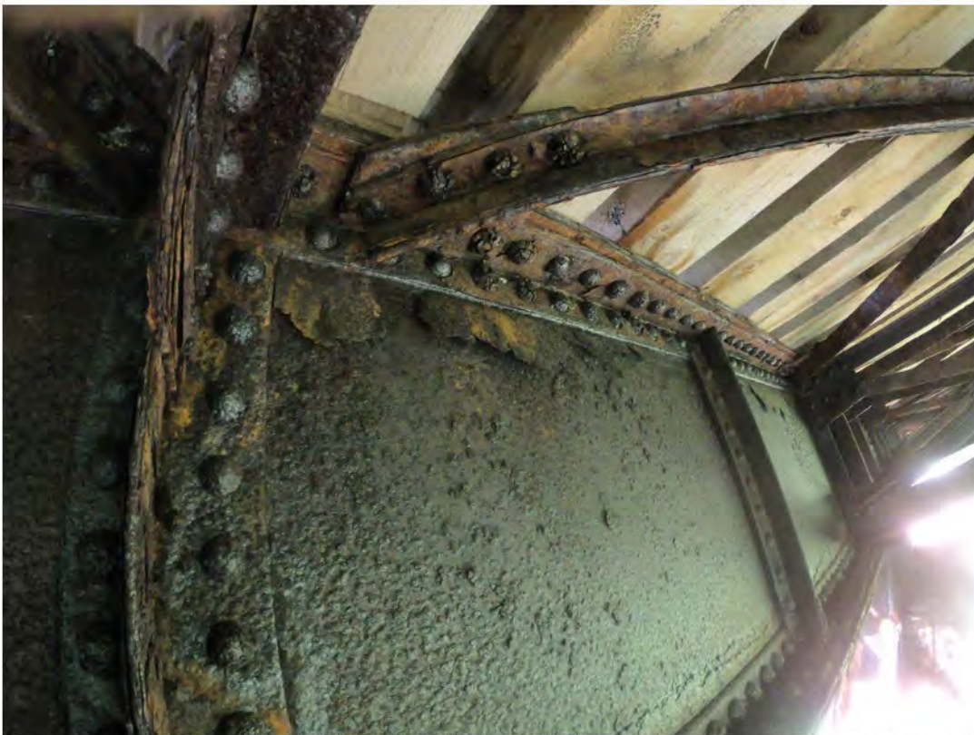
26. Medium Corrosion and Delamination on Girder at Soffit; Severe Corrosion of Lateral Bracing
