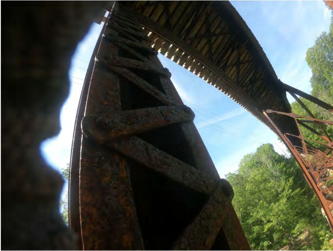
29. Severe Corrosion and Delamination on Column Bracing
