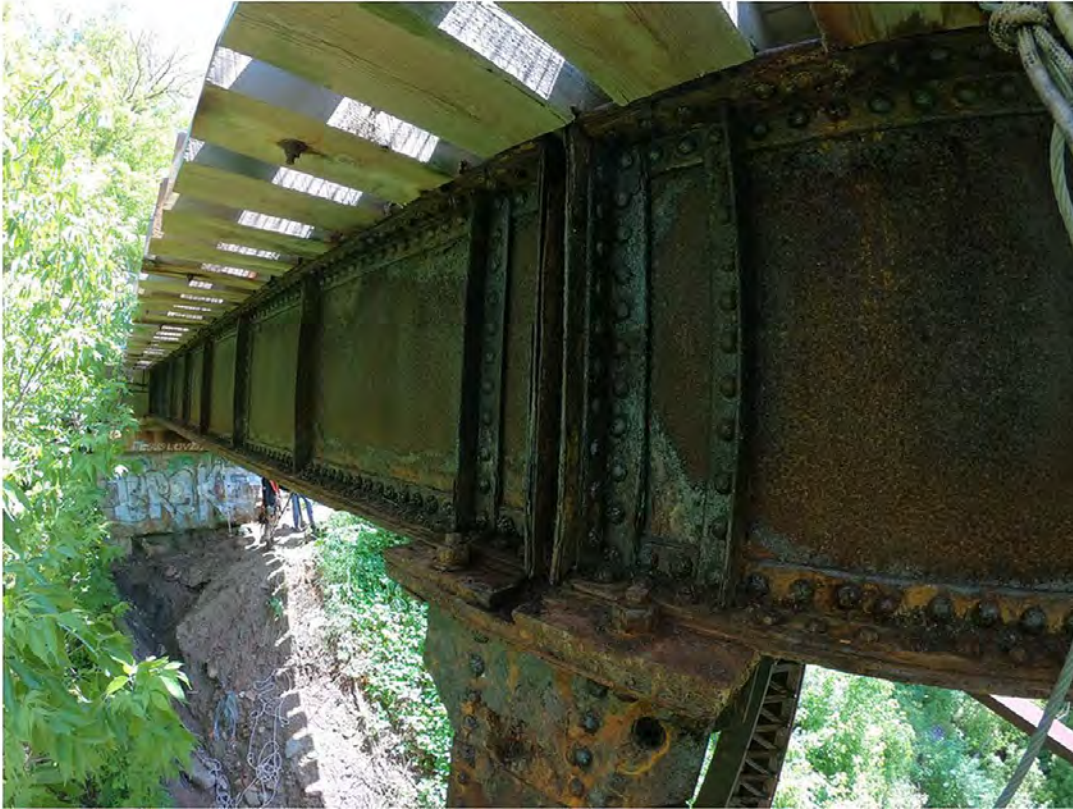
15. Severe Corrosion and Delamination on Girder
