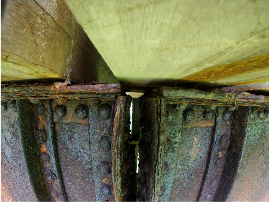
43. Very Severe Corrosion and Delamination at Ends of Girders Over Columns
