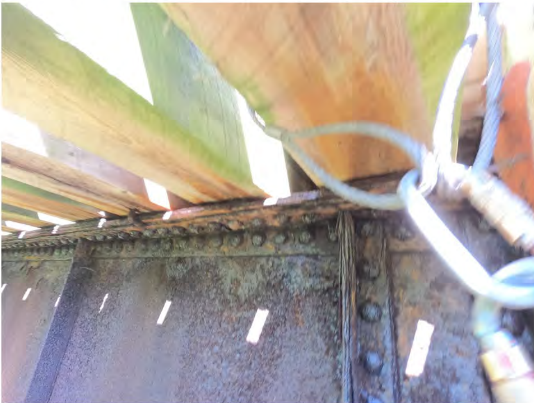
62. Severe Corrosion and Delamination of Web Stiffener
