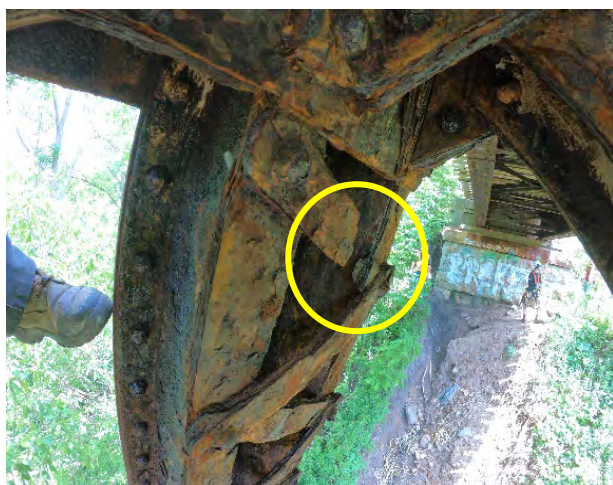
Figure 3 & 4: Severely Deteriorated Laces Bracing throughout, Note Broken Brace in Figure 3
