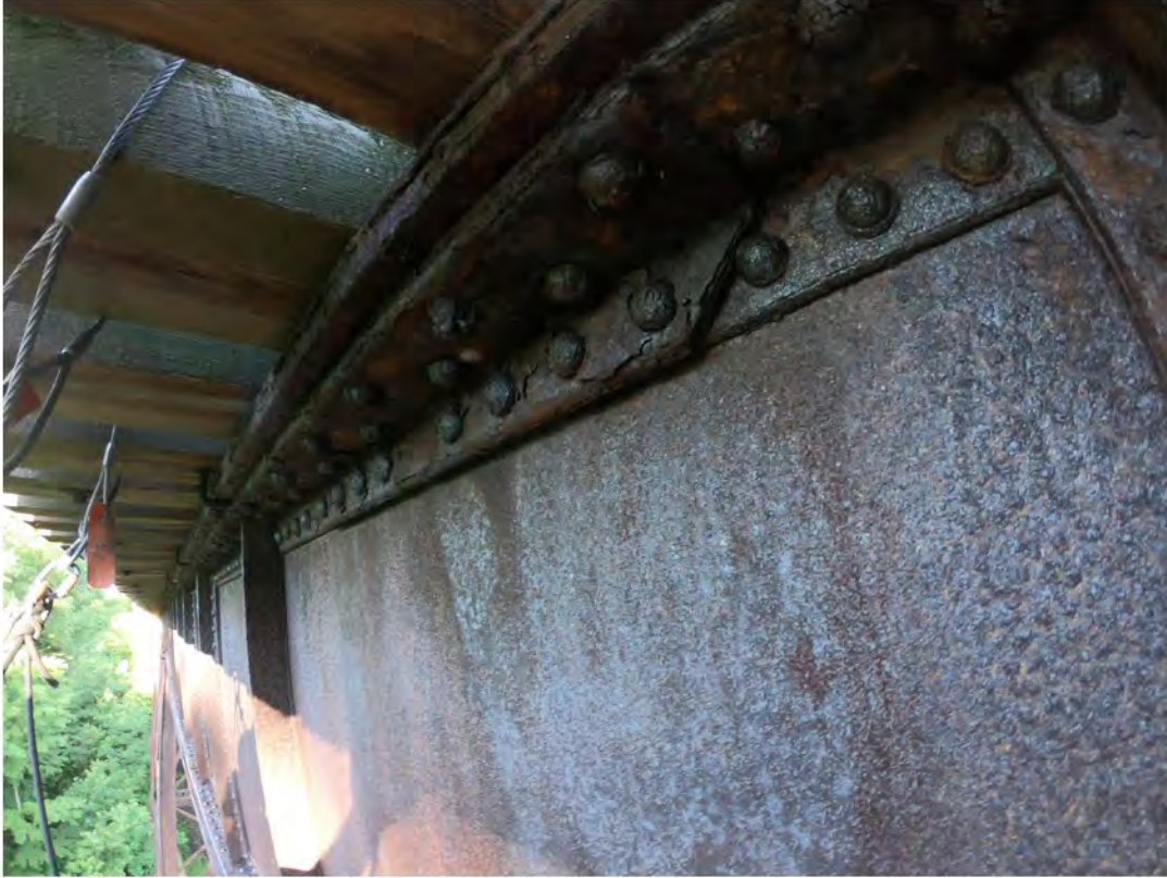
49. Severe Corrosion and Delamination of Angle Connections at the Top of Girder
