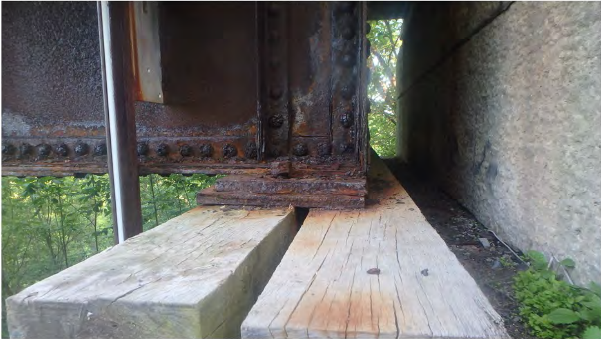
69. Medium Corrosion of Bearing Plate, and Severe Corrosion and Delamination of Girder End at East Abutment
