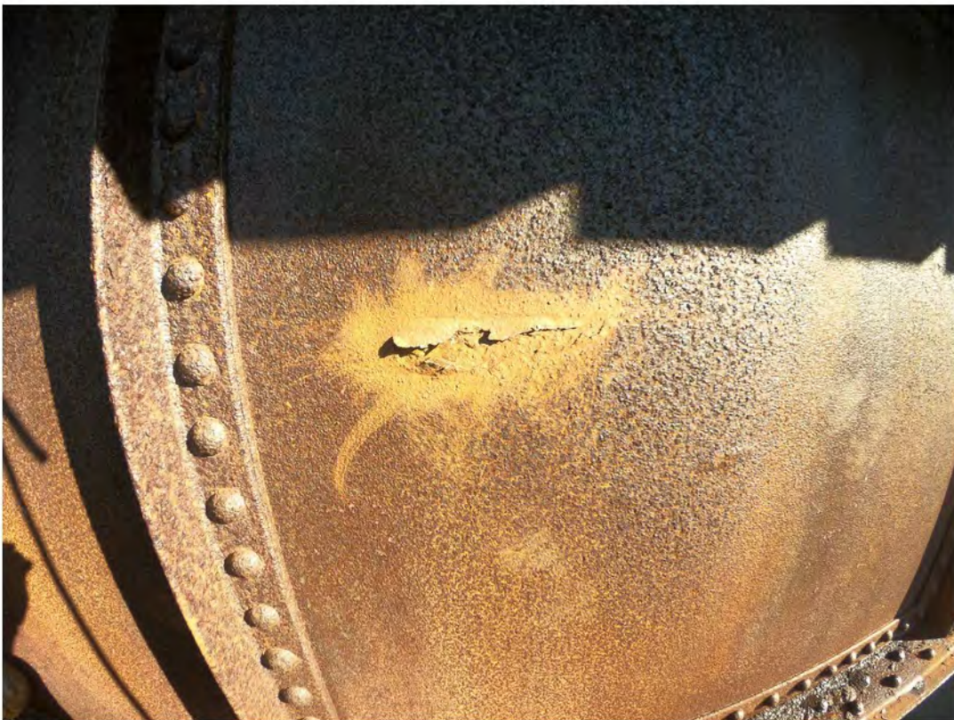
50. Localized Delamination on Exterior Face of Girder
