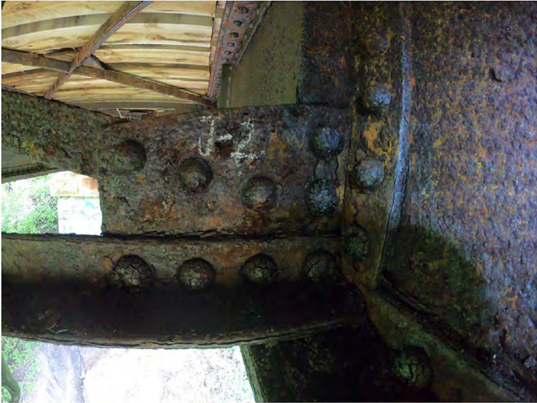
11. Medium Corrosion and Delamination of Diaphragm and Girder Connection
