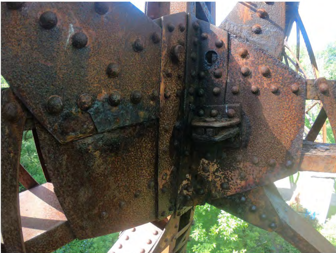
30. Medium Corrosion and Delamination of Connection at Middle of Column
