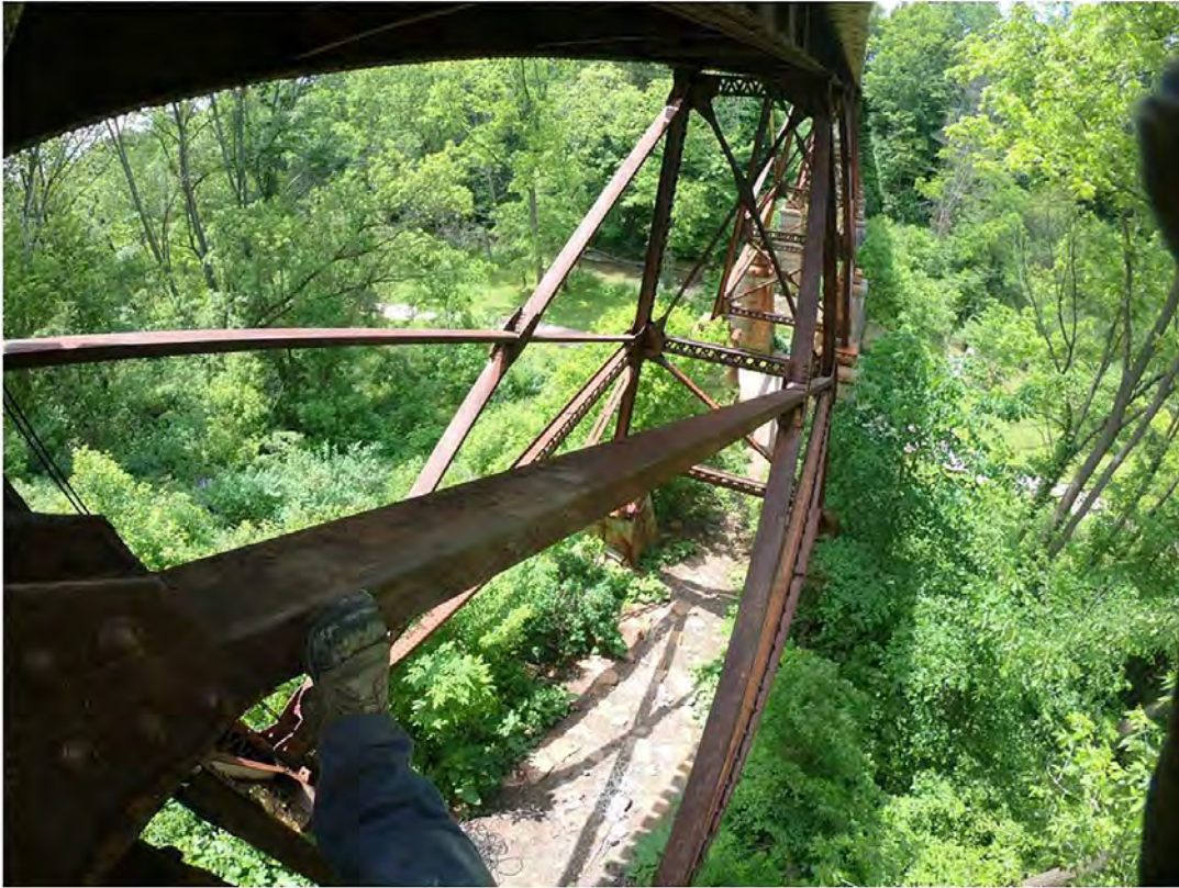
19. Surface Corrosion on Diagonal Bracing
