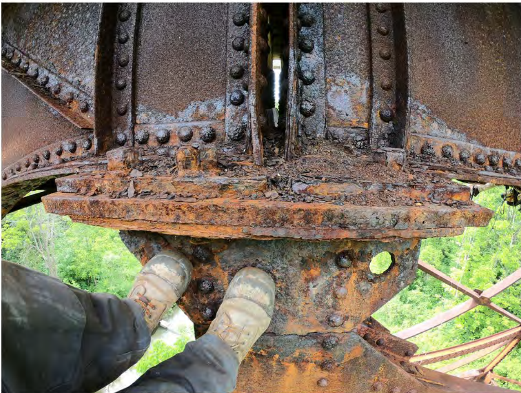
44. Severe Corrosion on Bottom Flange of Girder Resting on Bearing Plate; Medium Corrosion and Delamination of Bearing Plate
