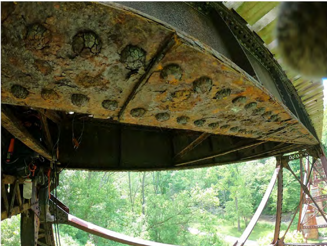
22. Medium Corrosion, Delamination, and Cracking of Rivets at Connection Plates on Girder
