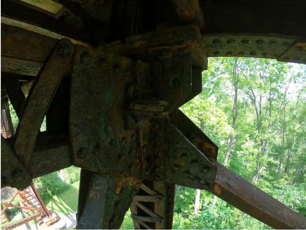
39. Severe Deterioration and Delamination at Connection of Girder, Column, and Diagonal Bracing
