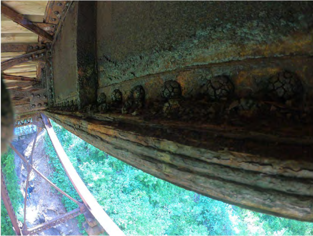
35. Severe Corrosion on Bottom Flange of Girder; Cracked Rivets
