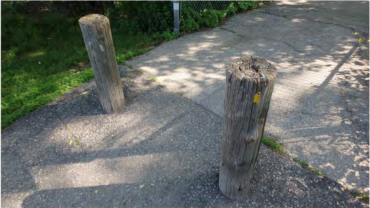
101. Checks and Splits in Wooden Posts at West Approach
