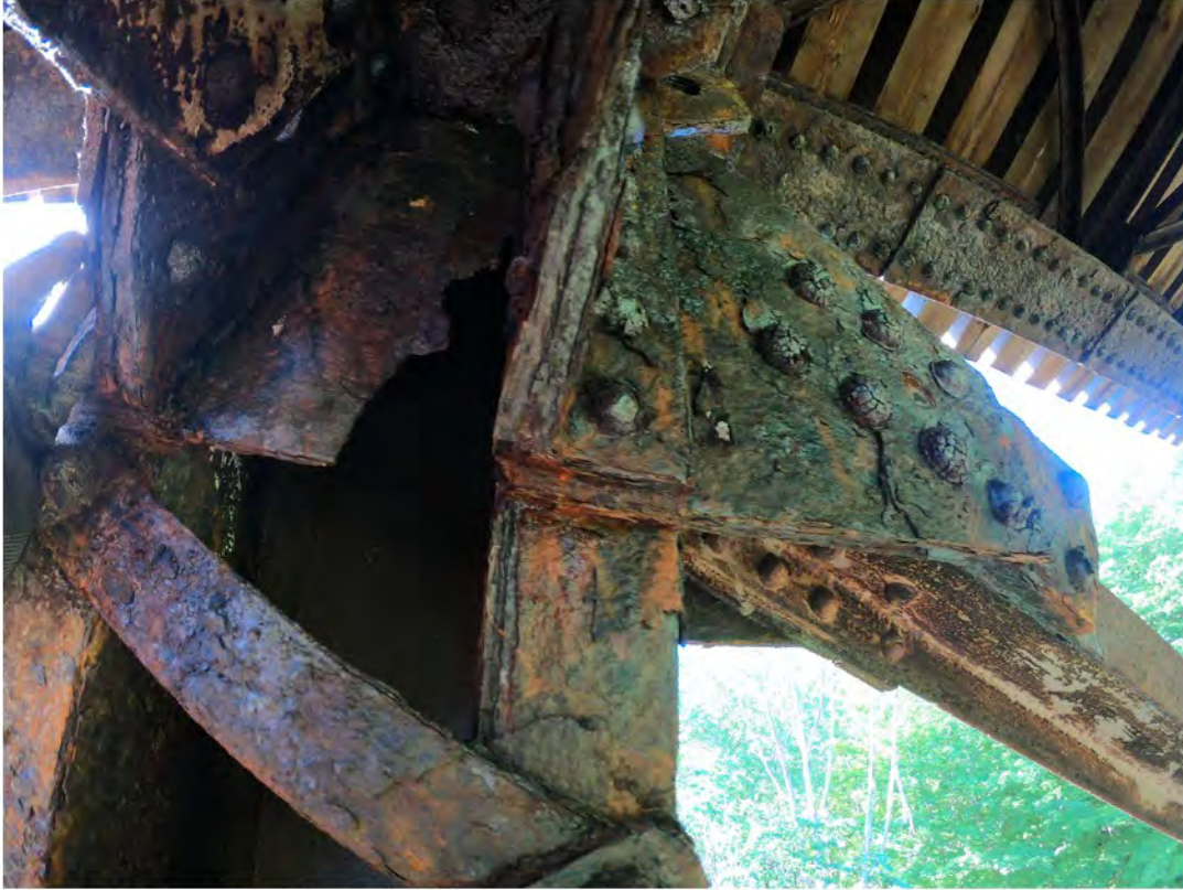
53. Very Severe Corrosion with Section Loss on Column Connection at South Column E
