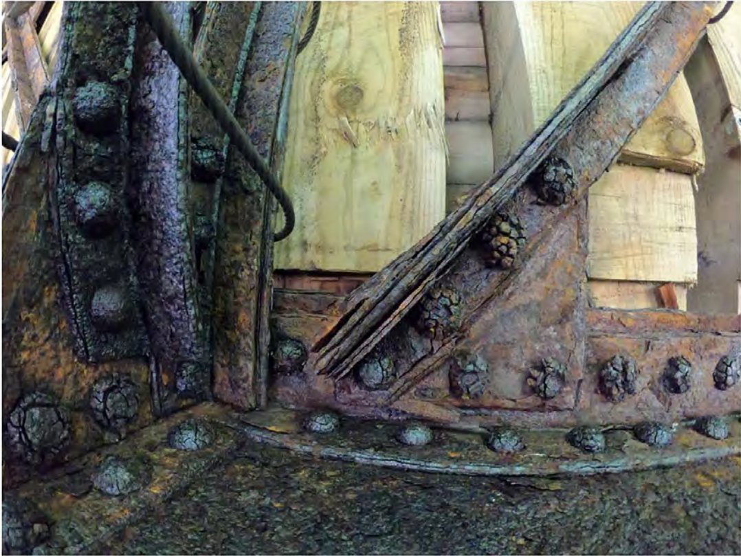
13. Severe Corrosion, Delamination, and Cracking of Rivets at Lateral Bracing and Girder
