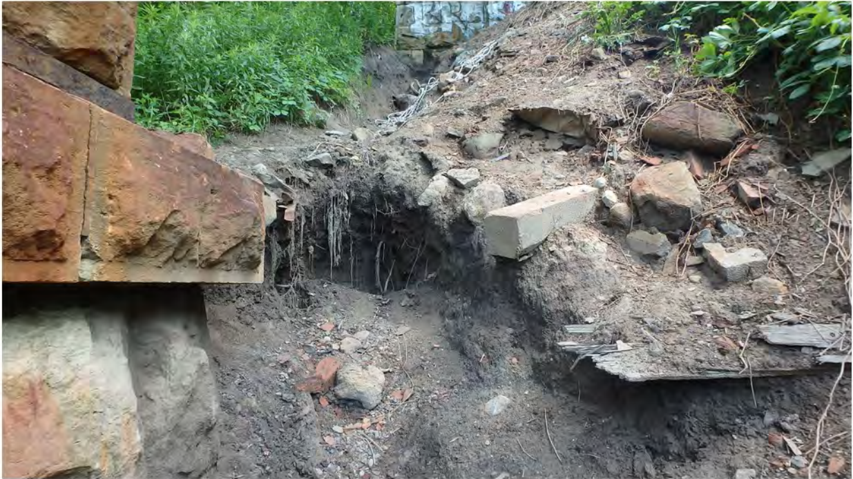
97. Severe Erosion From East Abutment Wall to North Pier
