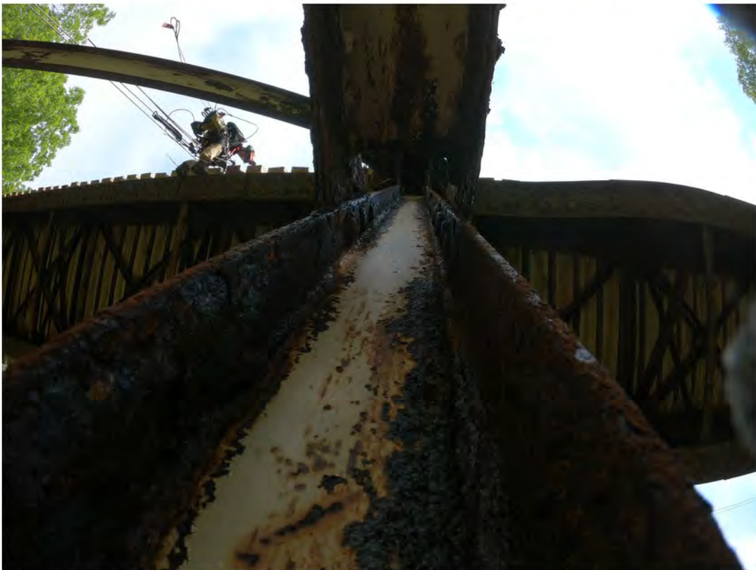
46. Severe Corrosion and Delamination on Both Flanges of Column
