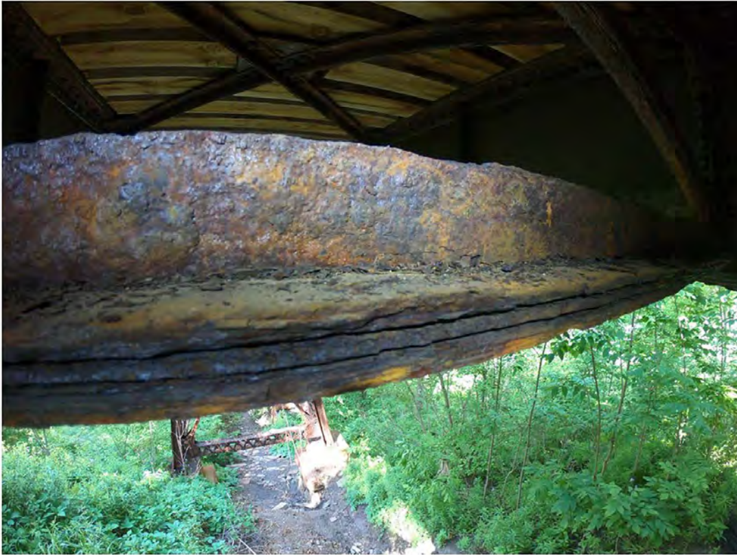
9. Severe Corrosion and Delamination on Horizontal Component of Diaphragm
