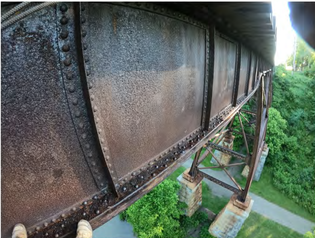
48. Medium Corrosion on Girder, Typical
