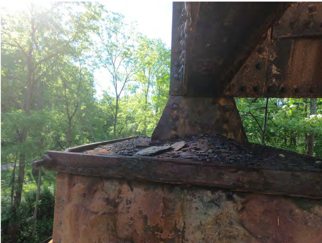
56. Severe Corrosion and Delamination of Column Bearing Connection
