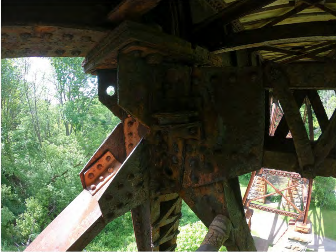
37. Very Severe Corrosion and Delamination at Column Connection to Girder; Separation of Bracing at Weld
