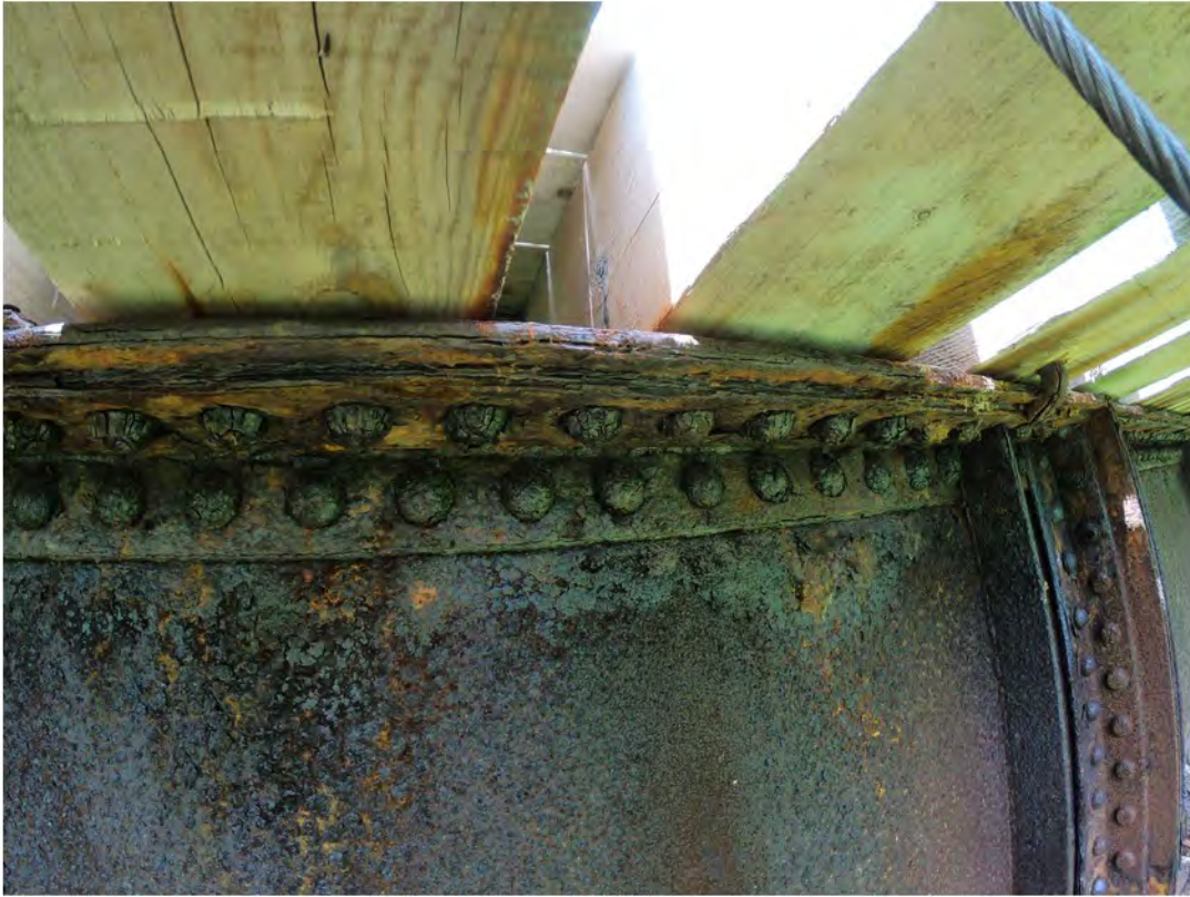
41. Severe Corrosion and Delamination on Top Flange of Girder
