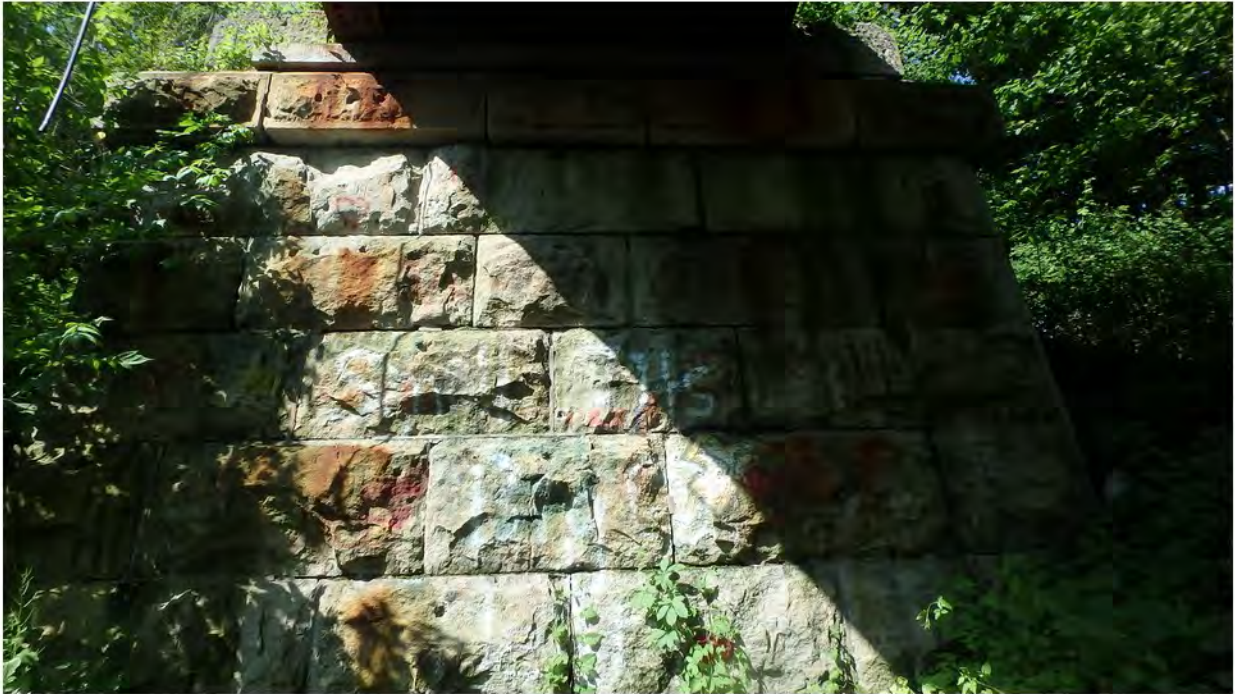
75. Minor Staining on West Abutment
