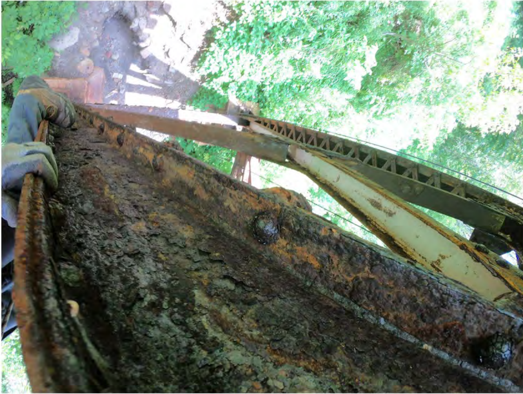
23. Severe Corrosion and Delamination of Column
