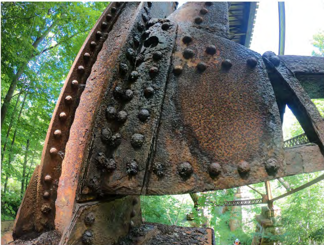
28. Very Severe Corrosion and Delamination at Connection of Column and Lateral Support
