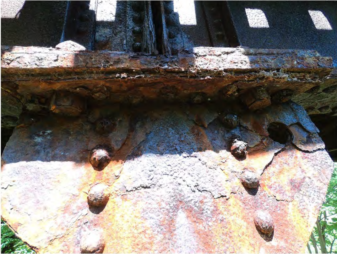
63. Severe Corrosion of Connection Plate and Bearing Plate at Connection Between Column and Girder
