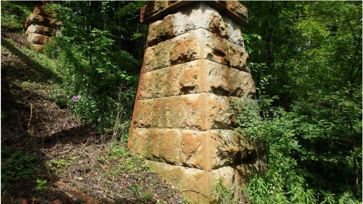
79. North C Pier; Staining Throughout
