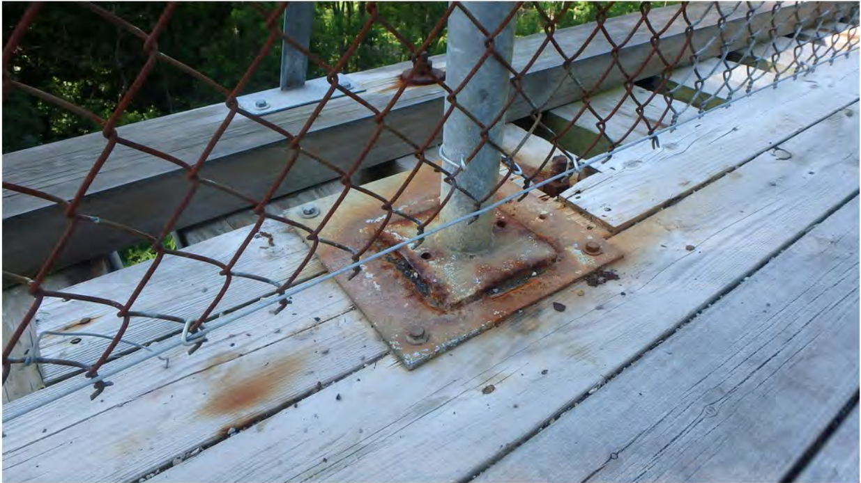
103. Medium Corrosion of Posts for Fencing on Bridge Deck
