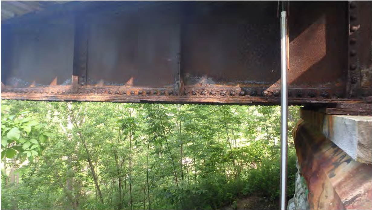
65. Severe Corrosion and Delamination of Angle at Bottom Flange of Girder
