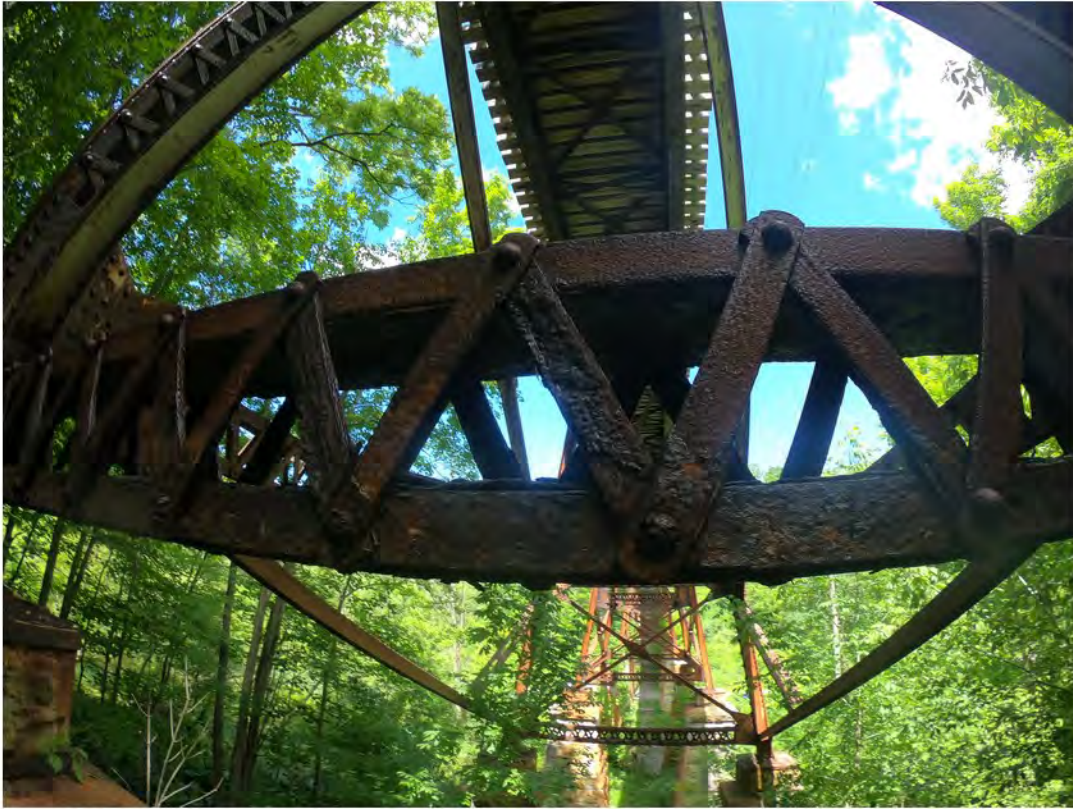
27. Very Severe Corrosion of Bracing on Lateral Support
