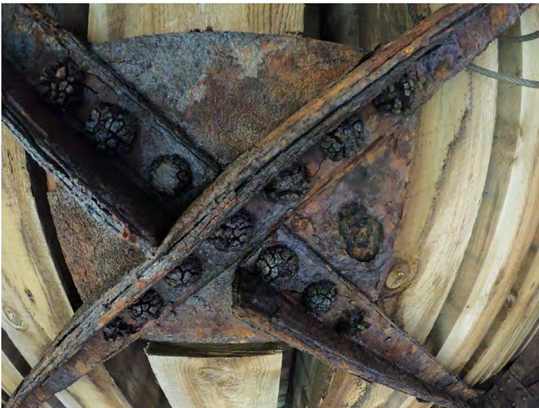
10. Severe Corrosion and Rivet Cracking on Lateral Bracing on Soffit
