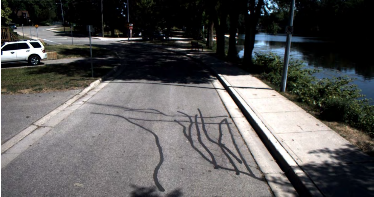
Pavement Condition Poor – PCI 40 – 57
