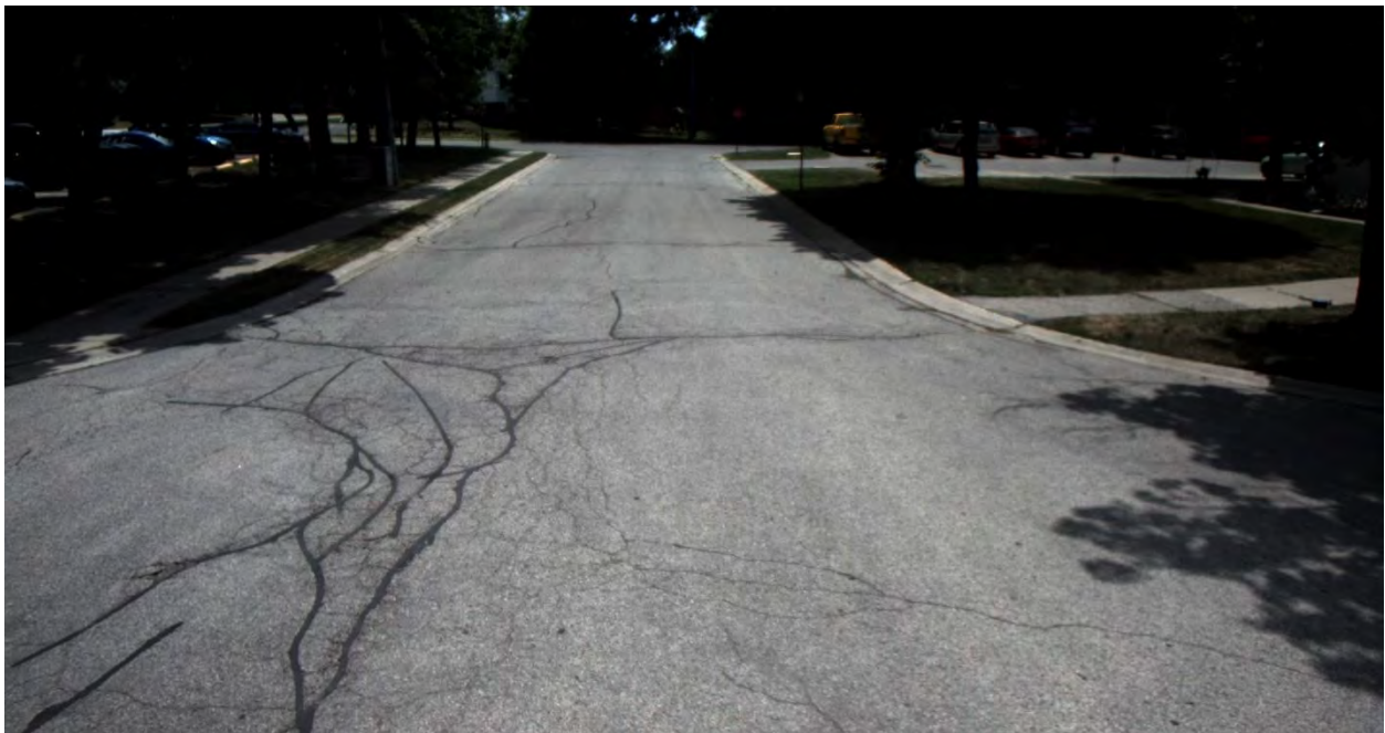
Pavement Condition Poor – PCI 40 – 57
