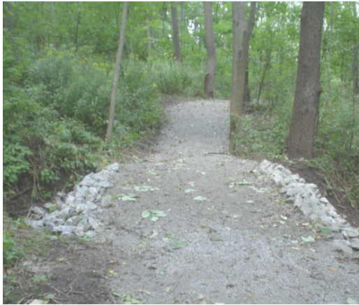
Infiltration trench and buried culvert
