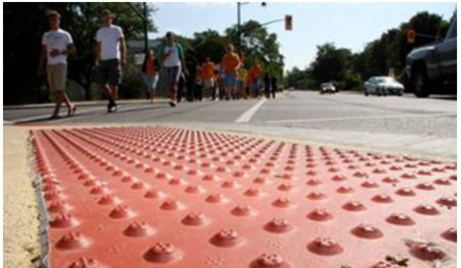
Textured surface at crosswalk. www.uwo.ca
